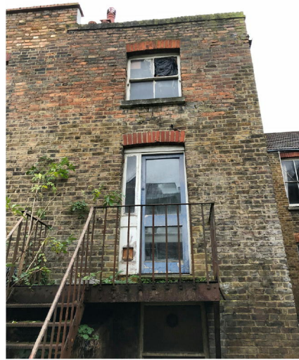
Fig.2 Photograph of rear elevation
