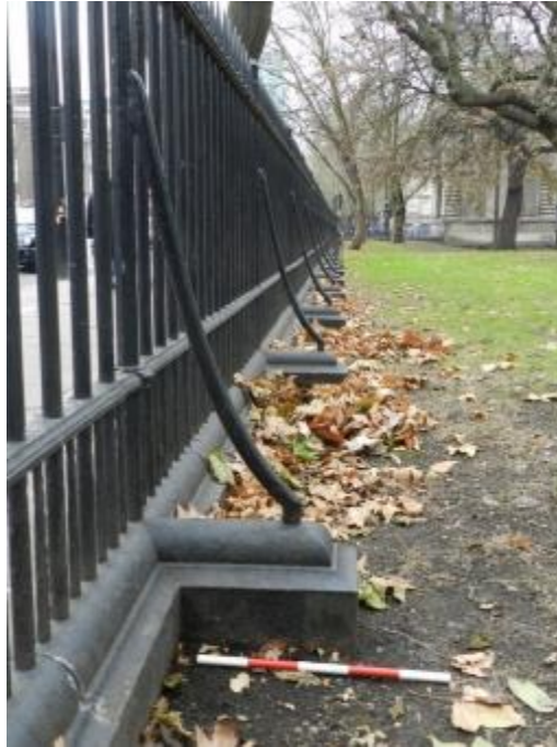
Figure 7 The rear of a backstay panel in the western group of railings, looking west
