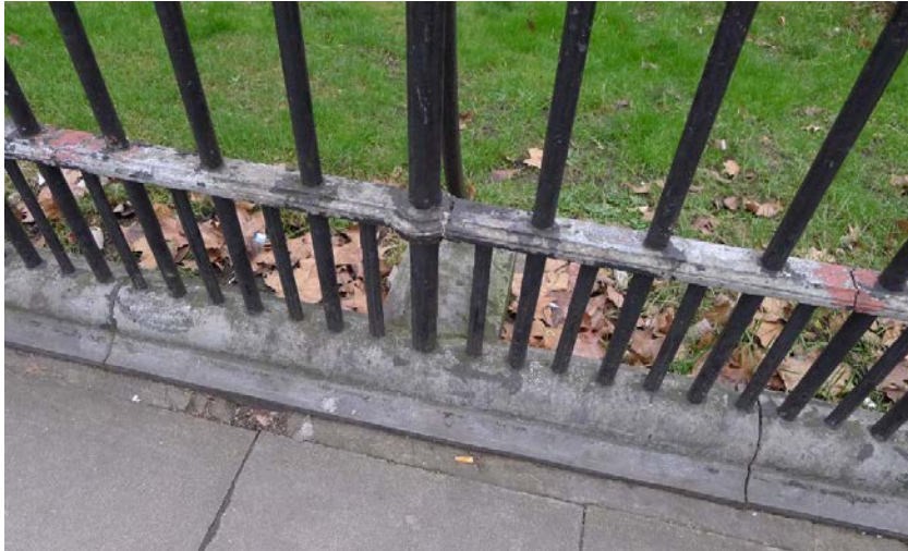
Figure 22 Fracture at the collar joint of the lower railing (around the principal, central paling).
