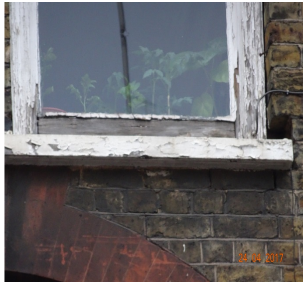
Second Floor Window
