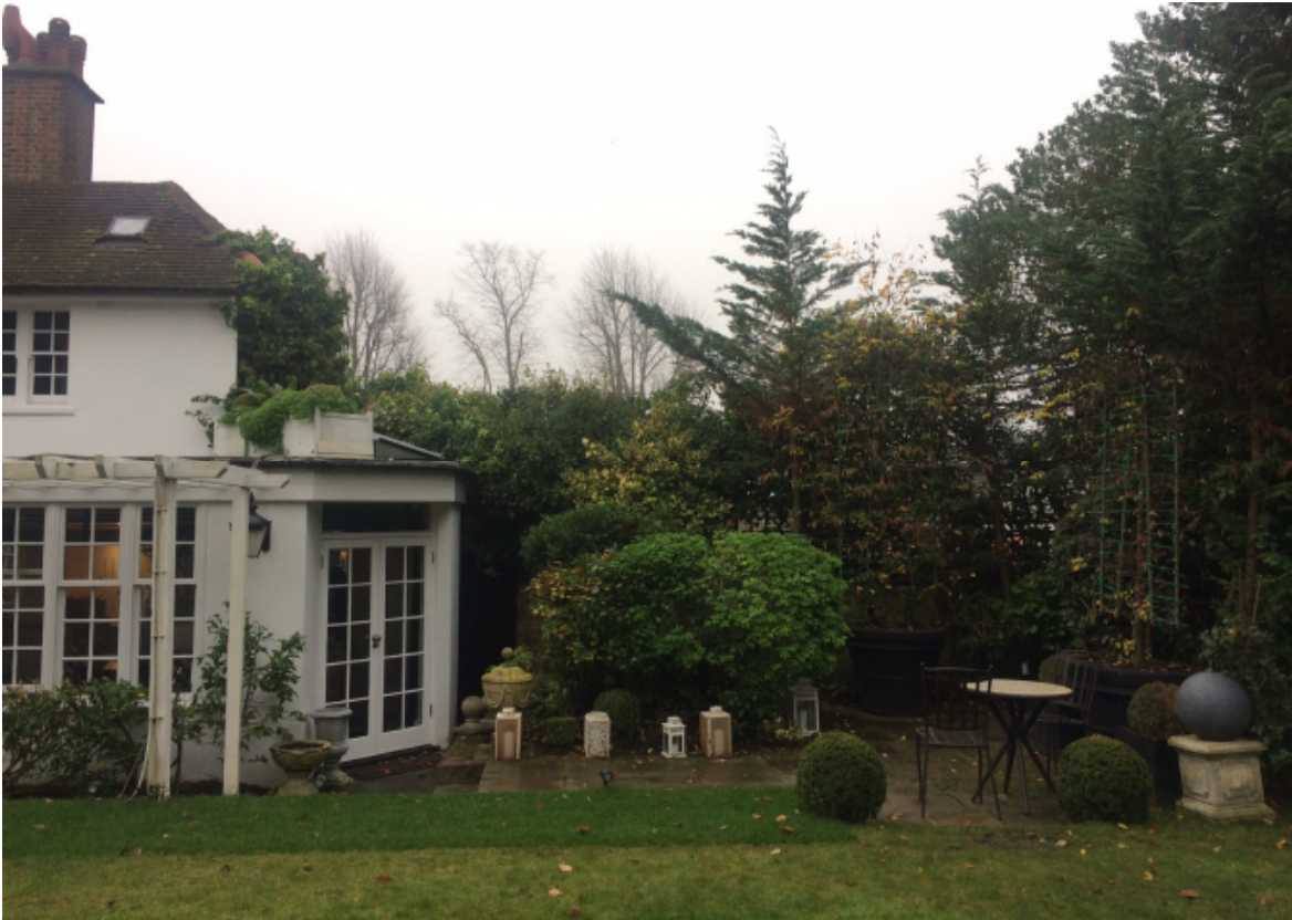
3. View towards area of the new extension.
