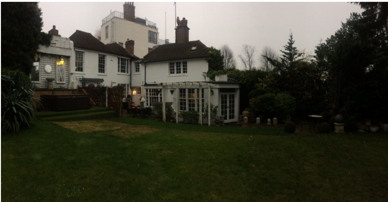
2. View from the garden – south east.
