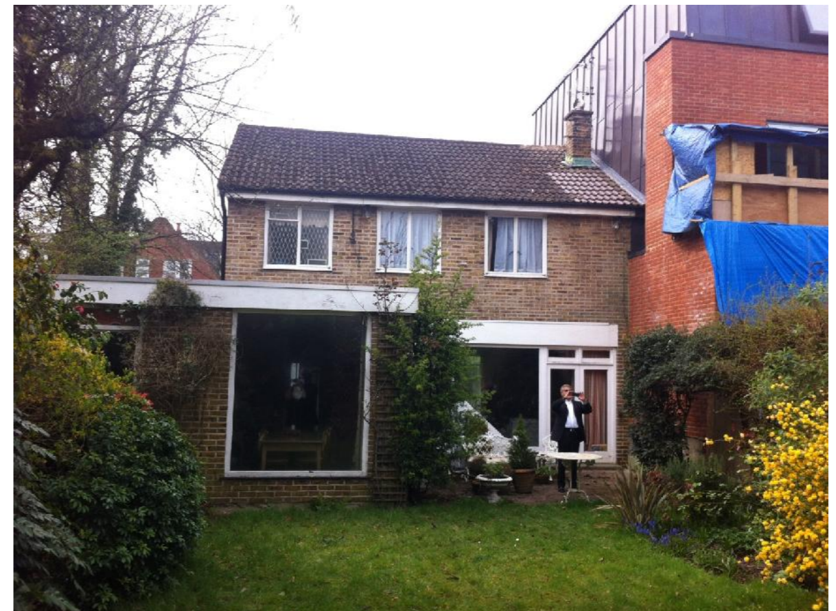
Fig. 3 Photograph from rear garden of existing property
