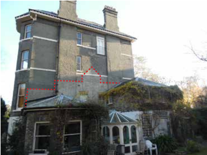
Garden View of Existing Extension. Original Extension evidenced through difference in brick colouration (as highlighted in red)
