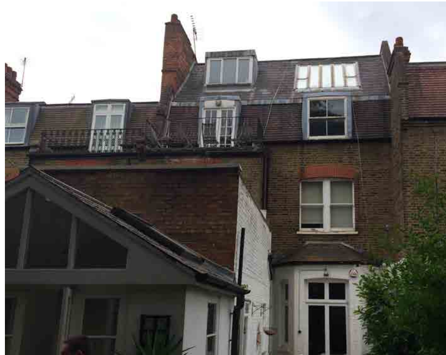
Rear facade to 190 Goldhurst Terrace with recent extension in foreground
