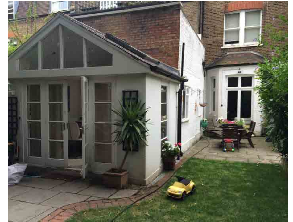
Rear facade to 190 Goldhurst Terrace with recent extension in foreground
