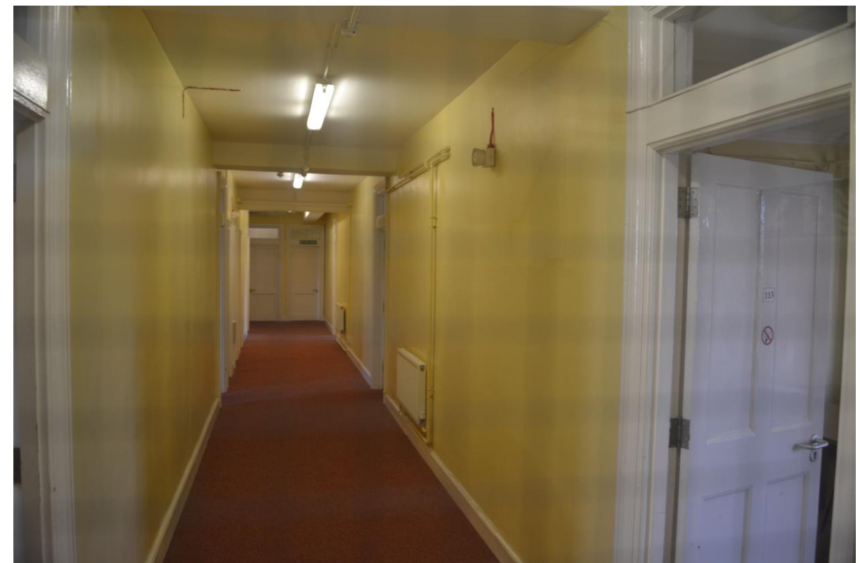
Figure 107 A photograph of the existing interiors at the upper floor levels of Bay House.
