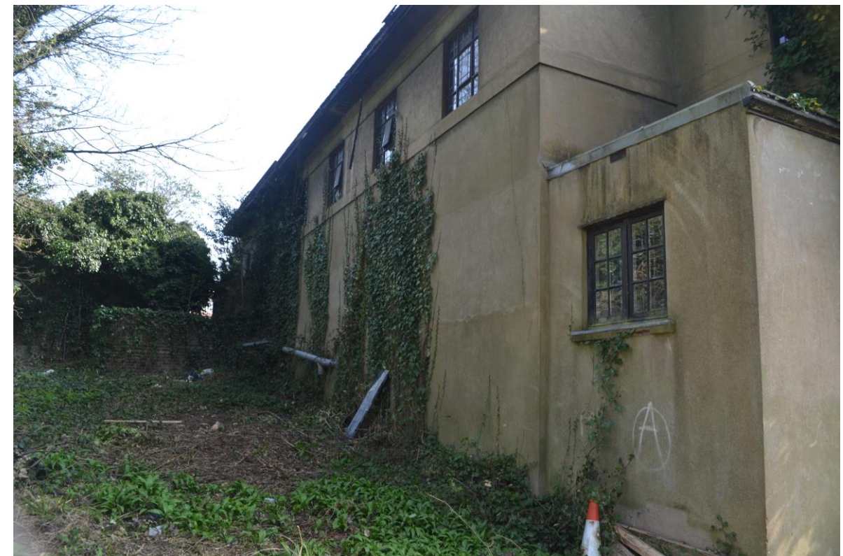
Figure 108. An image of the north elevation of the Chapel which is partially subsumed in the high ground level in this location.
