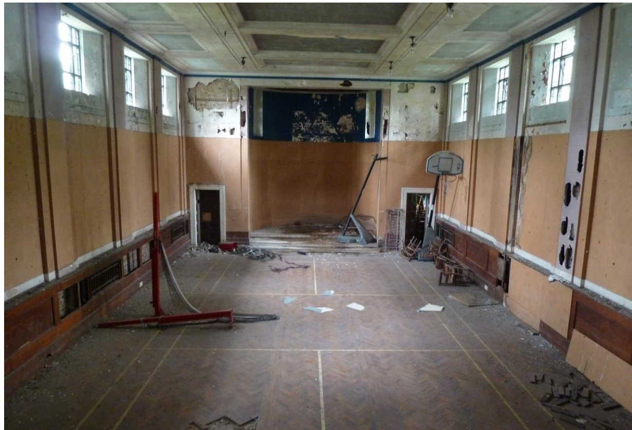
Figure 110. A view of the interior of the Chapel as seen from the entrance from the east elevation.
