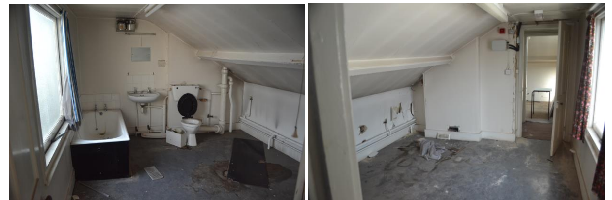
Figure 65. A photograph of a typical bathroom (left) and former bedroom (right) at the second floor level.
