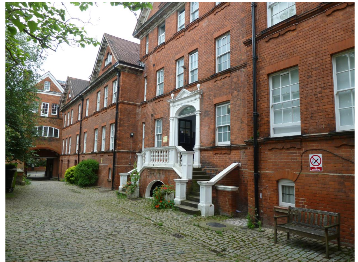
Figure 76 A photograph of the east elevation to the Maynard Wing photographed looking south with one's back to Lady Chapman Hall.
