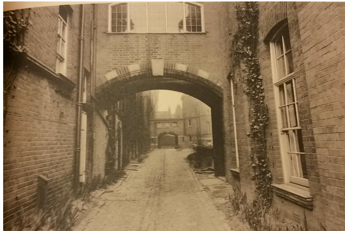
Figure 89. A photograph of the bridge structure which provided the original link between Skeel Library and Maynard Wing.
