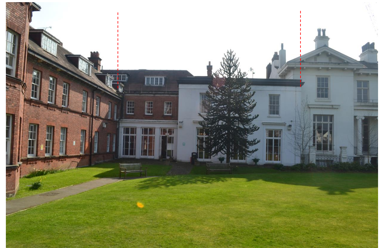
Figure 100 An image of the rear Bay House extension in its context with Kidderpore Hall and the Maynard Wing. The dotted red lines indicate the extent of the Bay House Lounge as seen from the rear from the garden.
