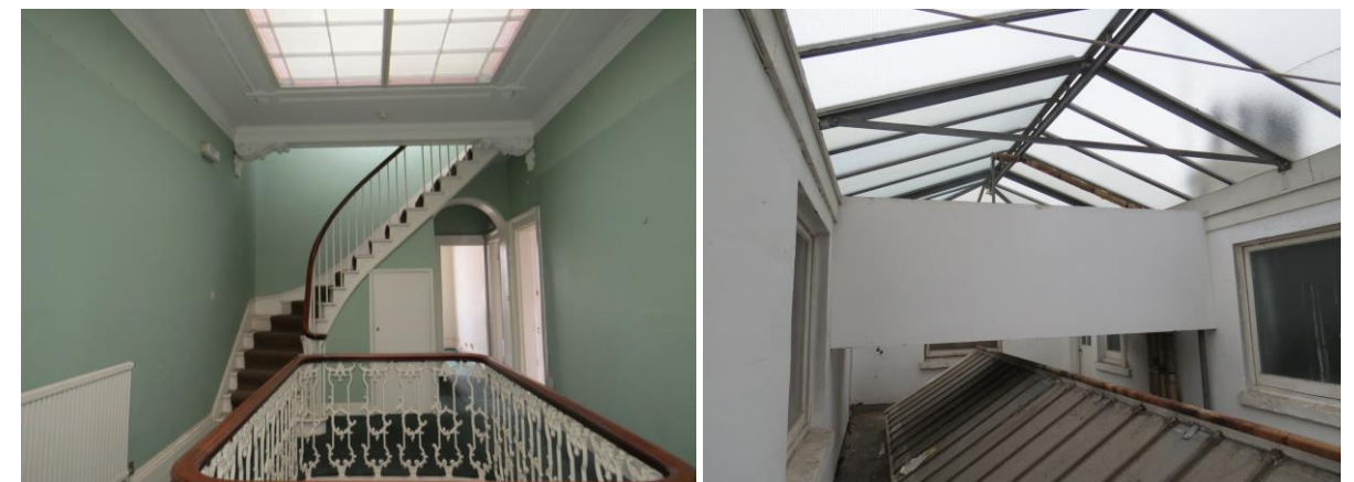
Figure 66. A photograph of the decorative skylight seen from a location on the first floor level landing, and the second floor level, and the structure located over the skylight at the second floor level.
