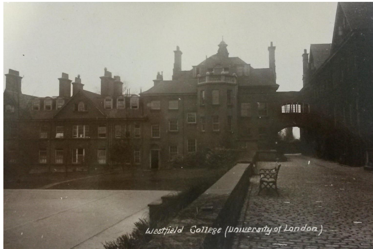
Figure 88 An image c.1905 showing the rear elevation of Skeel Library and the original bridge link between Skeel and Maynard.
