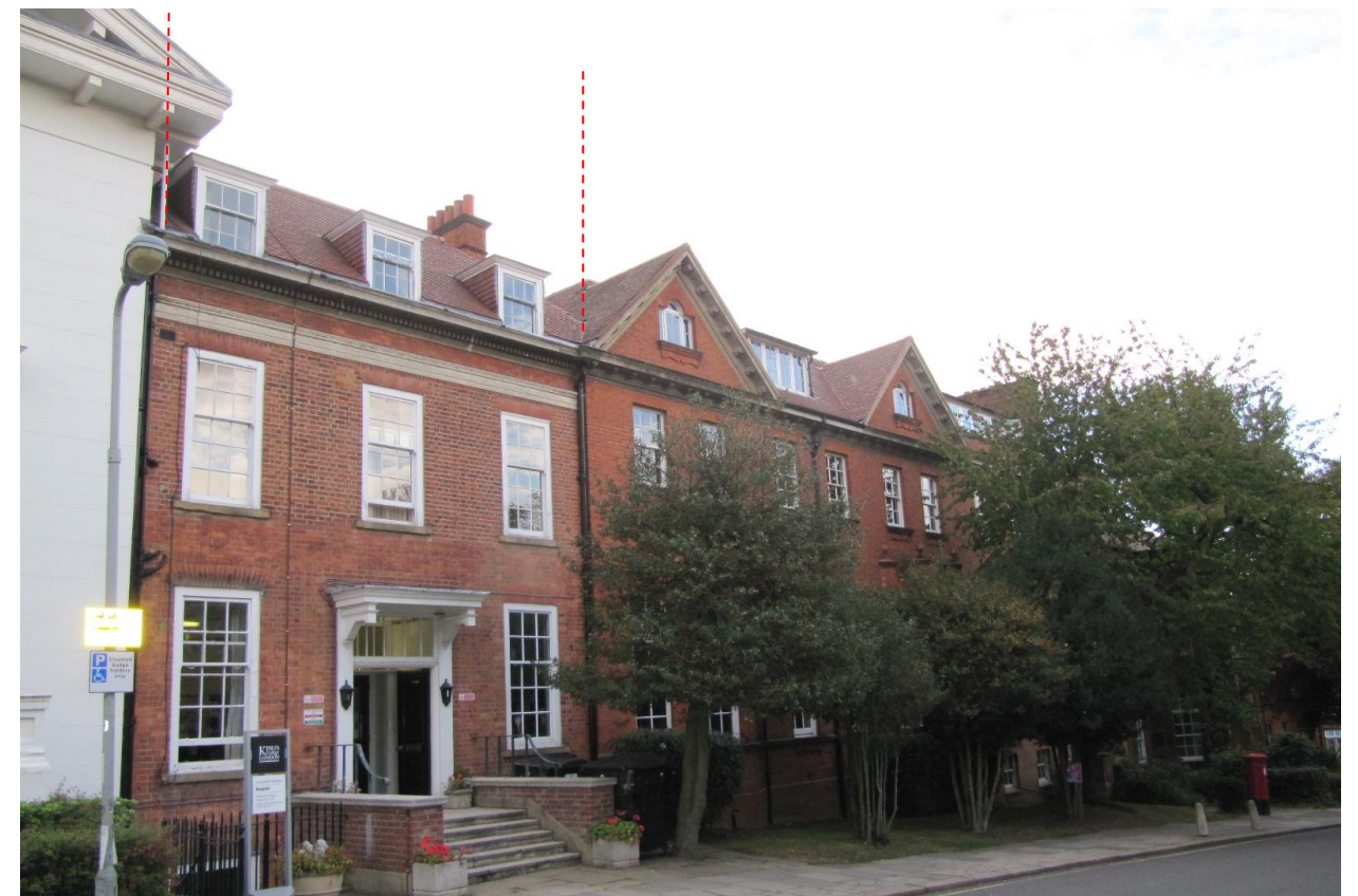
Figure 101. A photograph of the 1921 Bay House extension as seen from Kidderpore Avenue. The red dotted lines are indicative of the extent of the Bay House infill.
