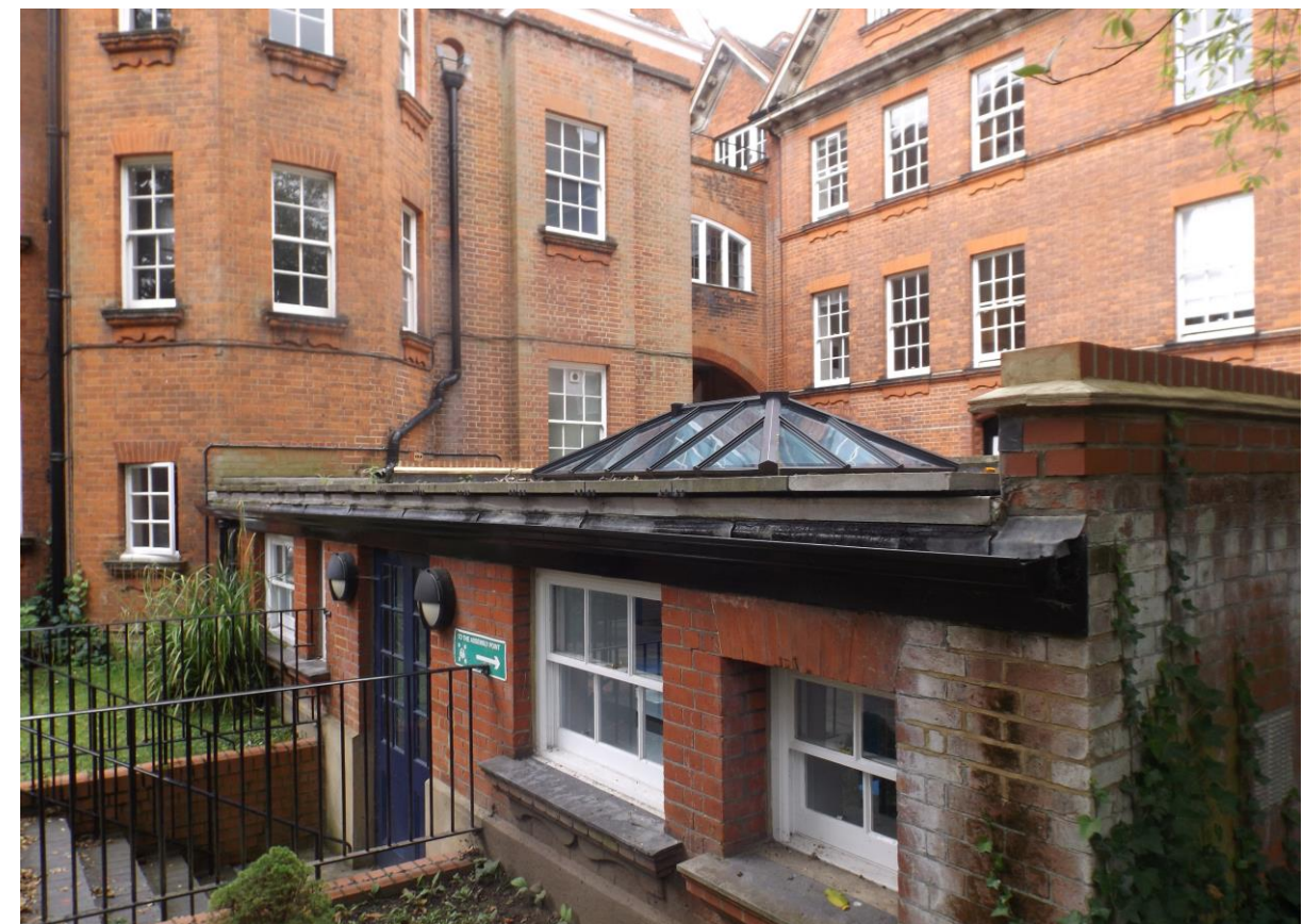
Figure 91. The single storey extension to the rear of the former Skeel Library.
