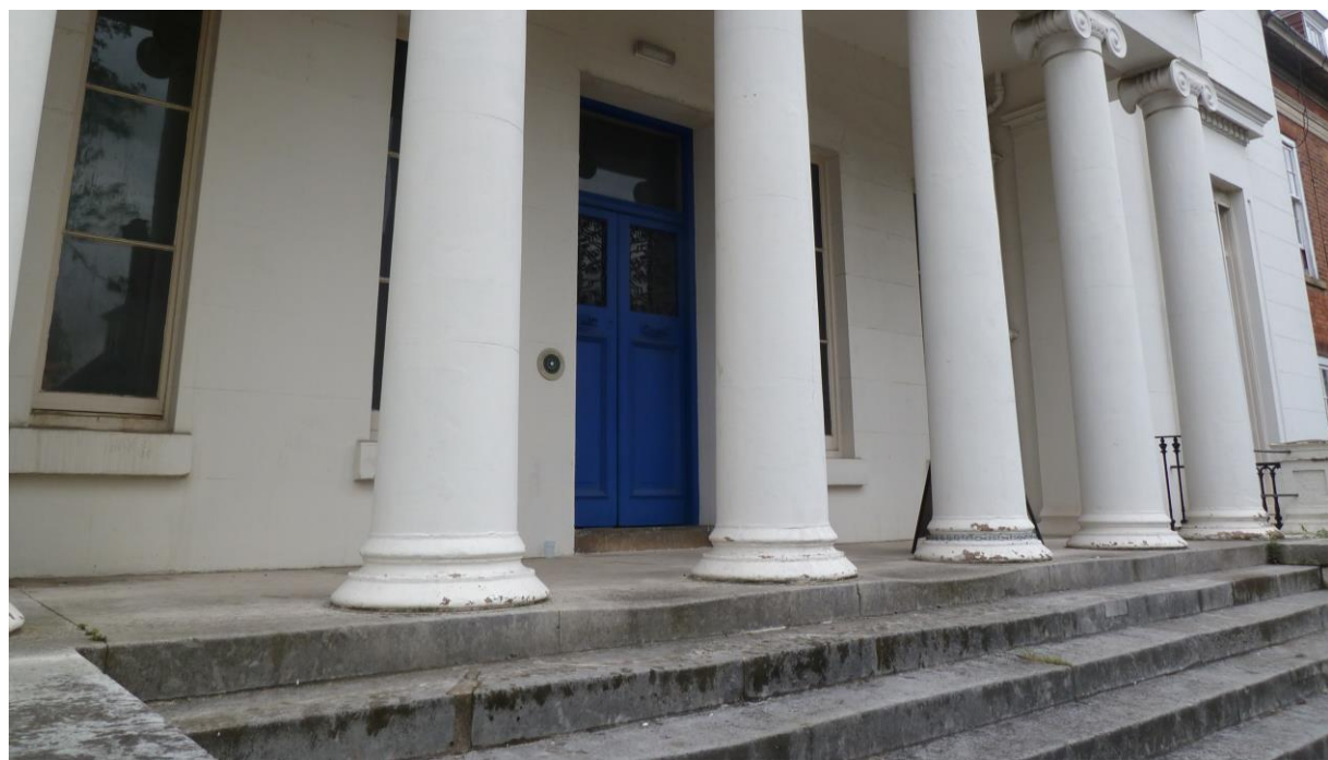
Figure 54 The entrance steps to Kidderpore Hall accessed from Kidderpore Avenue. The plaster render and the stonework of the steps are in need of refurbishment.
