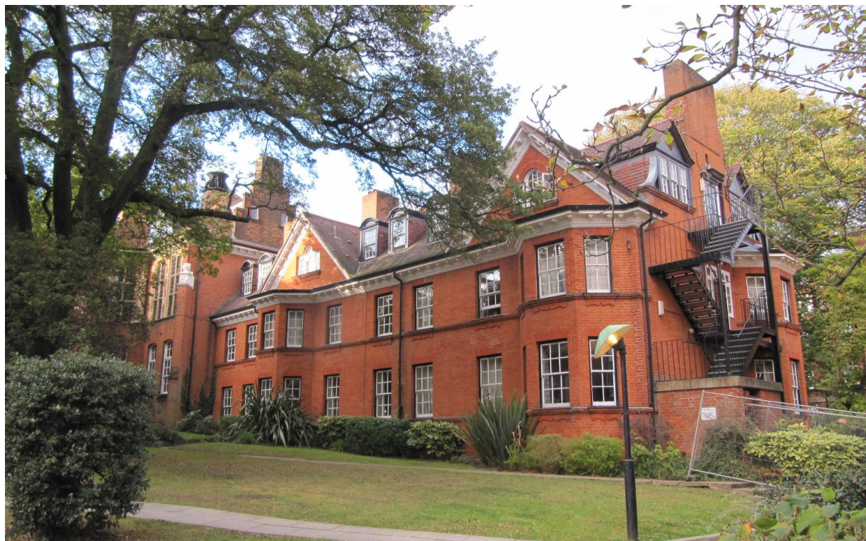
Figure 16 A photograph of the principal elevation of Dudin Brown as seen from Kidderpore Avenue.
