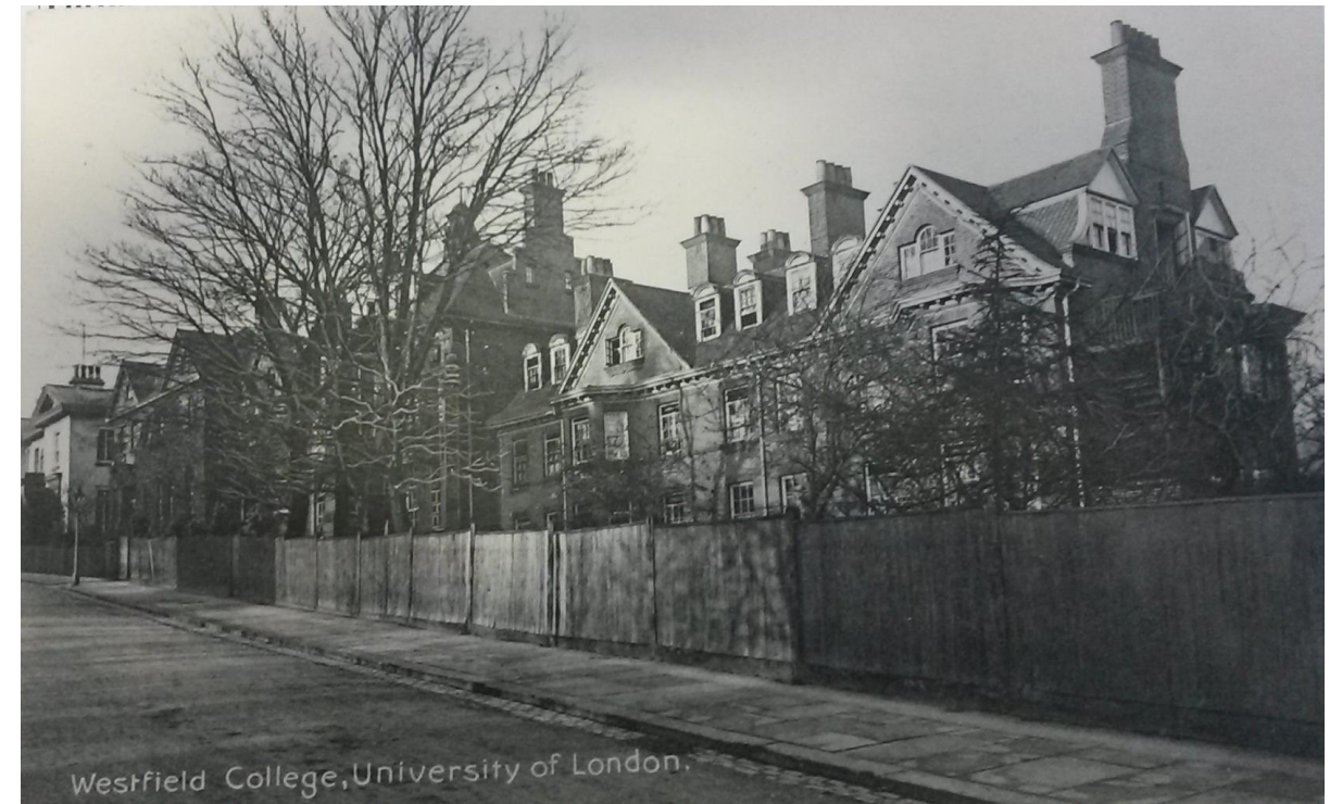
Figure 29. An early photograph of Dudin Brown as seen from Kidderpore Avenue looking north, with Kidderpore Hall seen in the background.
