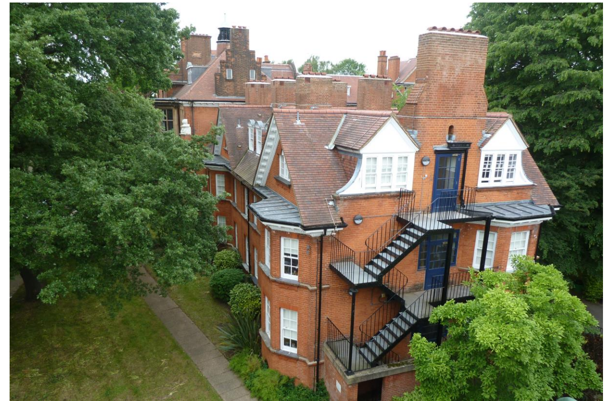
Figure 33 An aerial view showing the later addition of the fire escape staircase.
