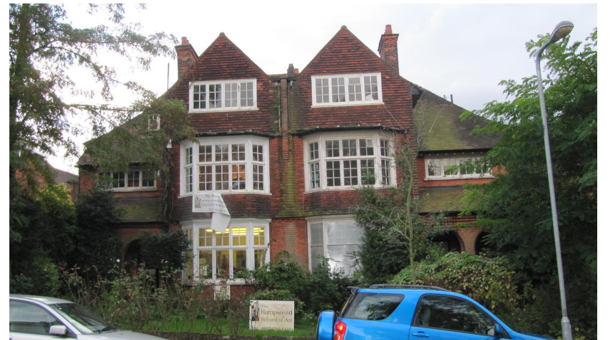
Figure 27 Typical semi-detached former dwellings within the Redington Froggnal Conservation Area.
