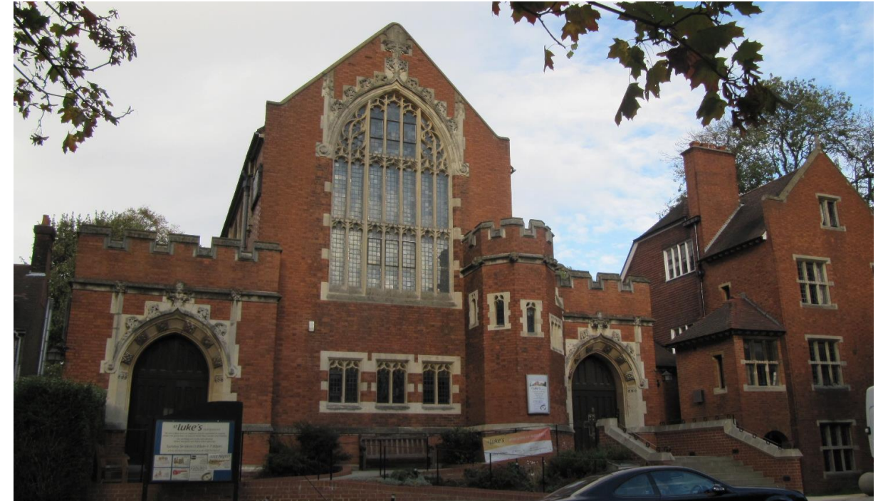
Figure 26 A photograph of the Grade II* listed Church at St Luke's which is situated to the west of the application site. The Grade II listed Vicarage is seen to the right of this photograph.
