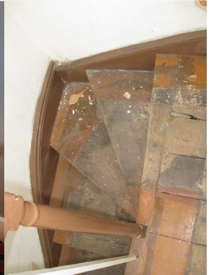
Newel post 2 nd floor landing
