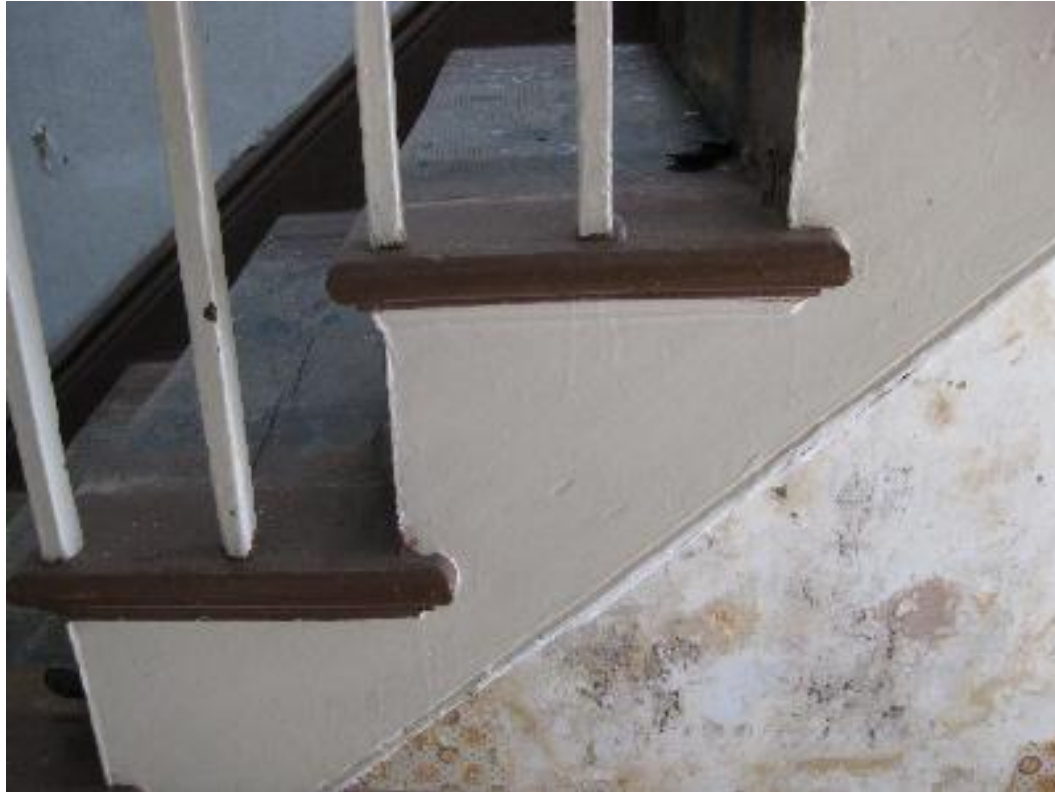
Detail of open string and stick balusters
