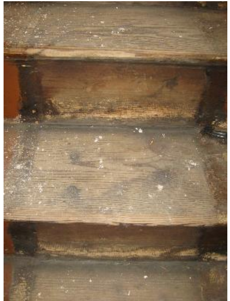
Detail of stair treads
