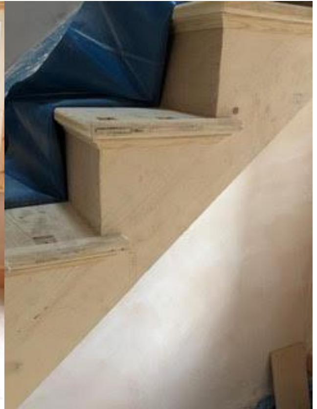
Detail of moulding to treads
