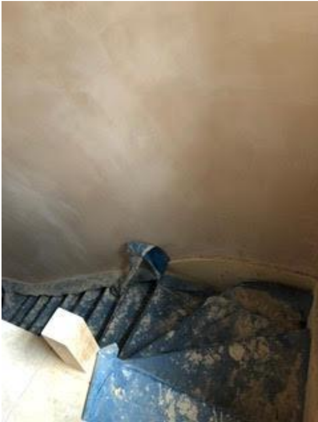
2 nd floor landing
