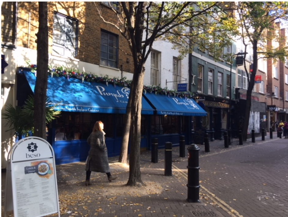
Photo 6 (above): Shopfront of No. 82 Neal Street adjacent to No. 192
