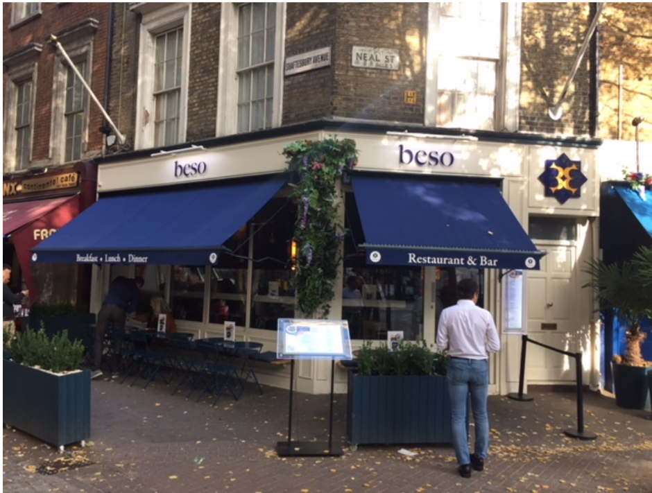
Photo 1 (above): Shopfront and fascia signage at 190 Shaftesbury Avenue as installed
