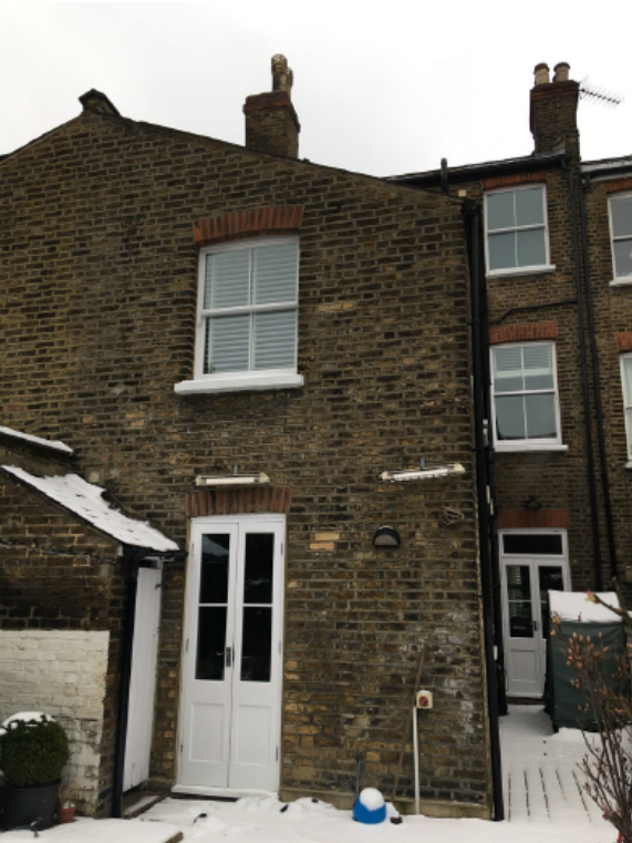
Photo 4 – Rear elevation of no.69 Roderick Road
