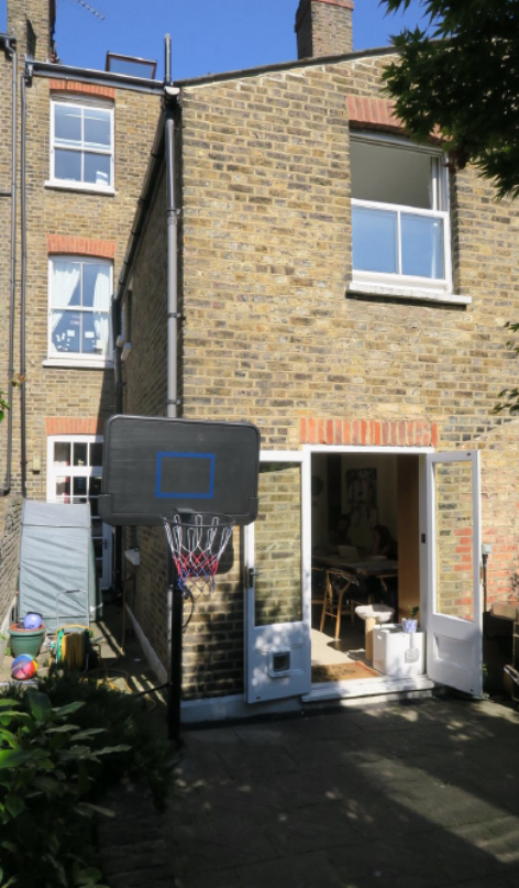
Photo 3 – rear elevation of no.67 Roderick Road
