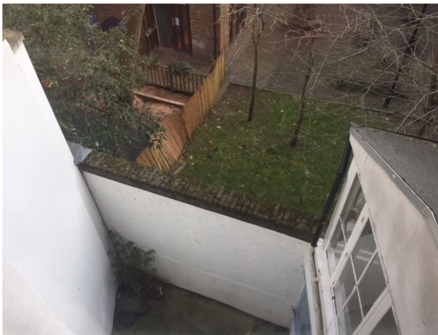
Photo 4: Rear external terrace area viewed from upper floors
