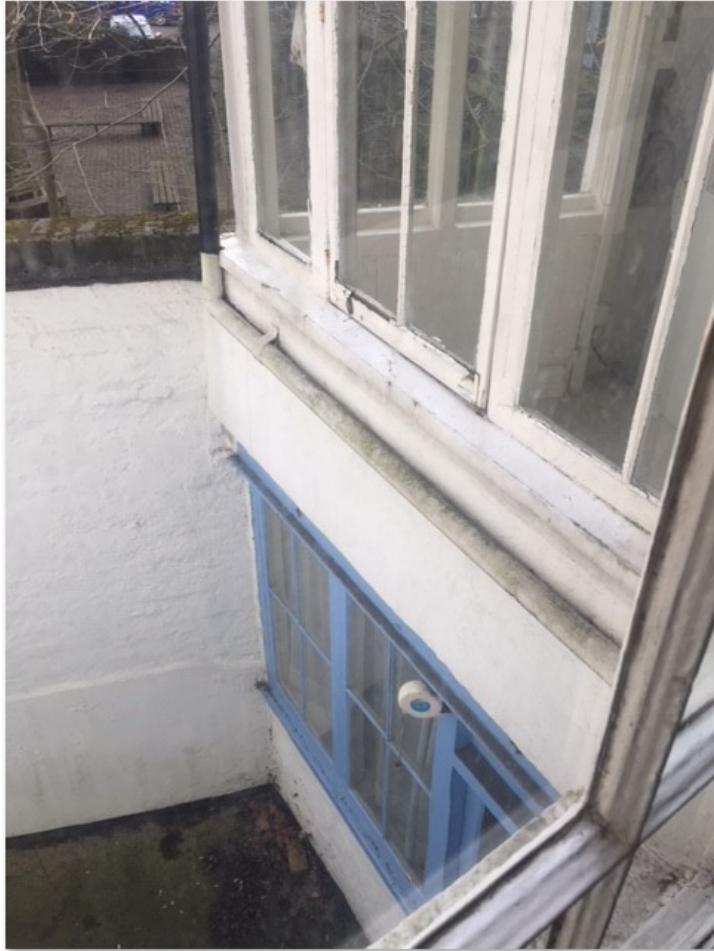
Photo 3: Existing two storey rear extension
