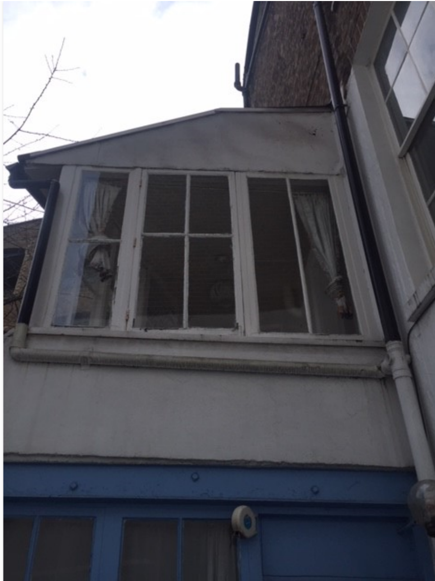
Photo 5: Existing rear extension viewed from external courtyard
