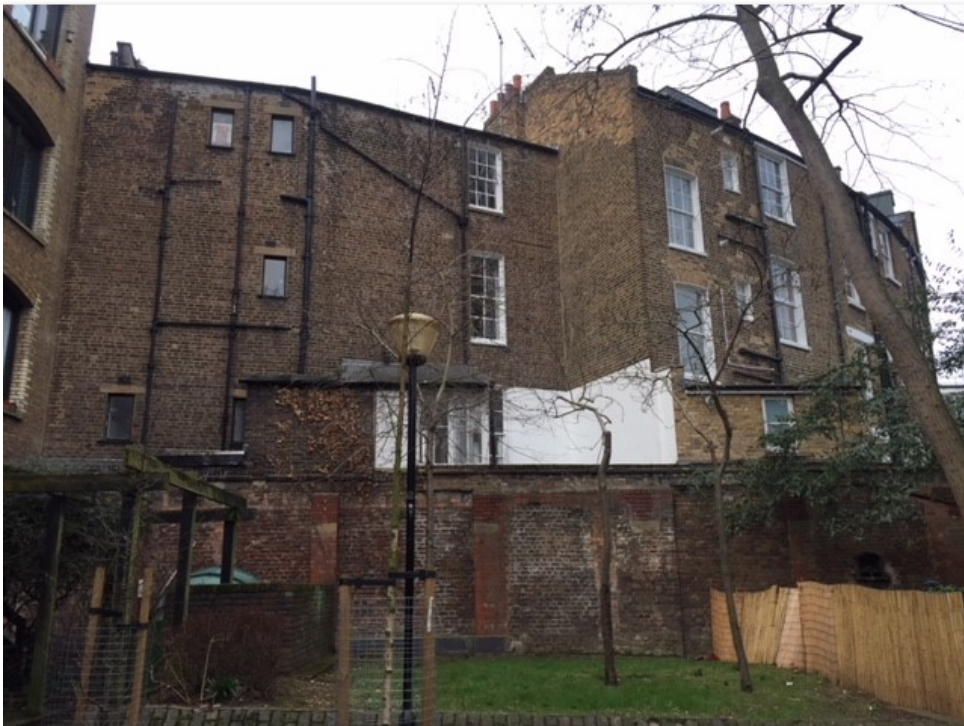
Photo 2: Rear elevation viewed from Hopkinson's Place to the rear
