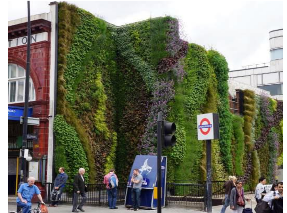
Edgware Road Tube Station, London
