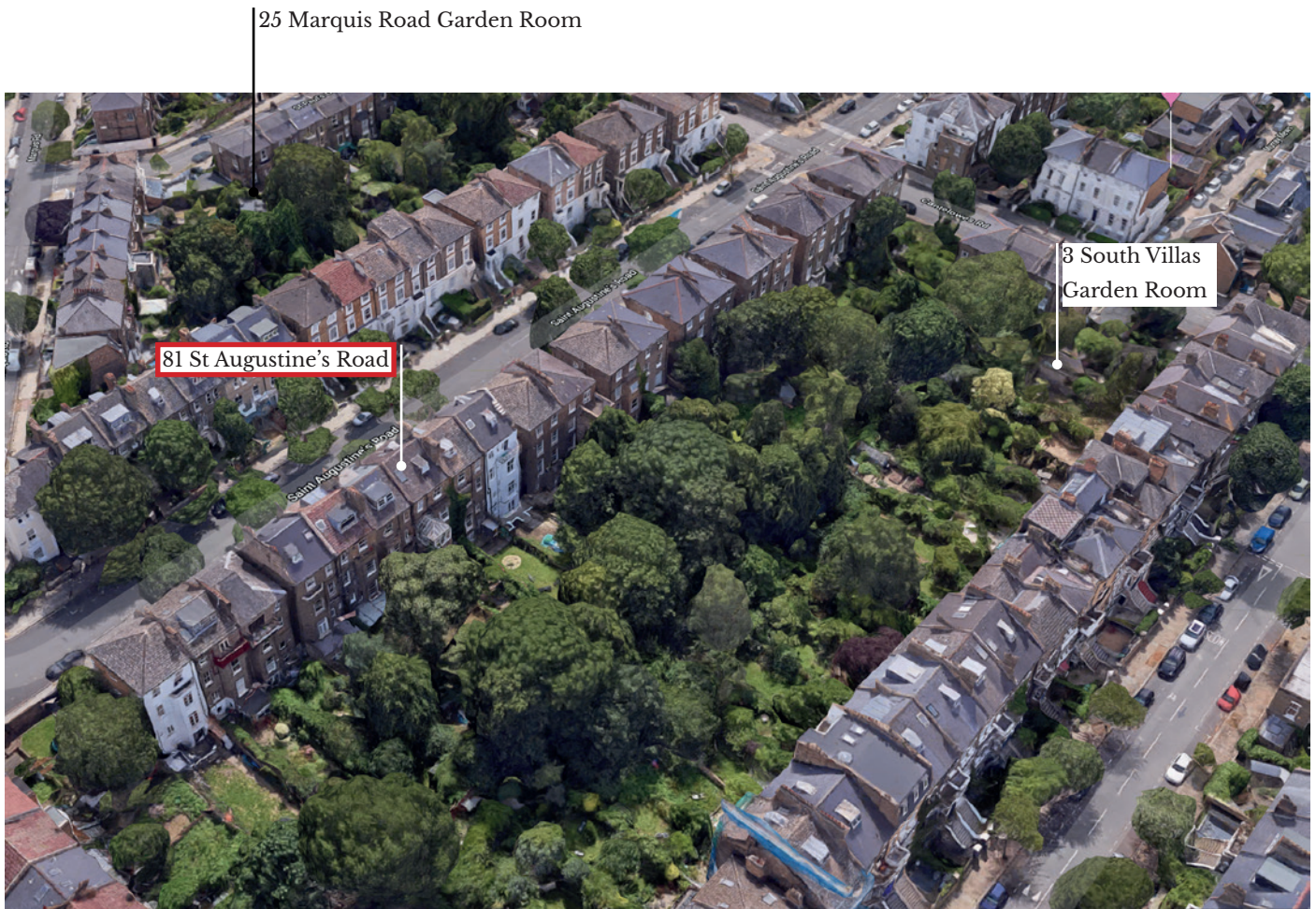
Aerial view of St Augustine's Road and South Villas gardens.
