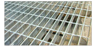
Example of galvanized steel mesh walkway
