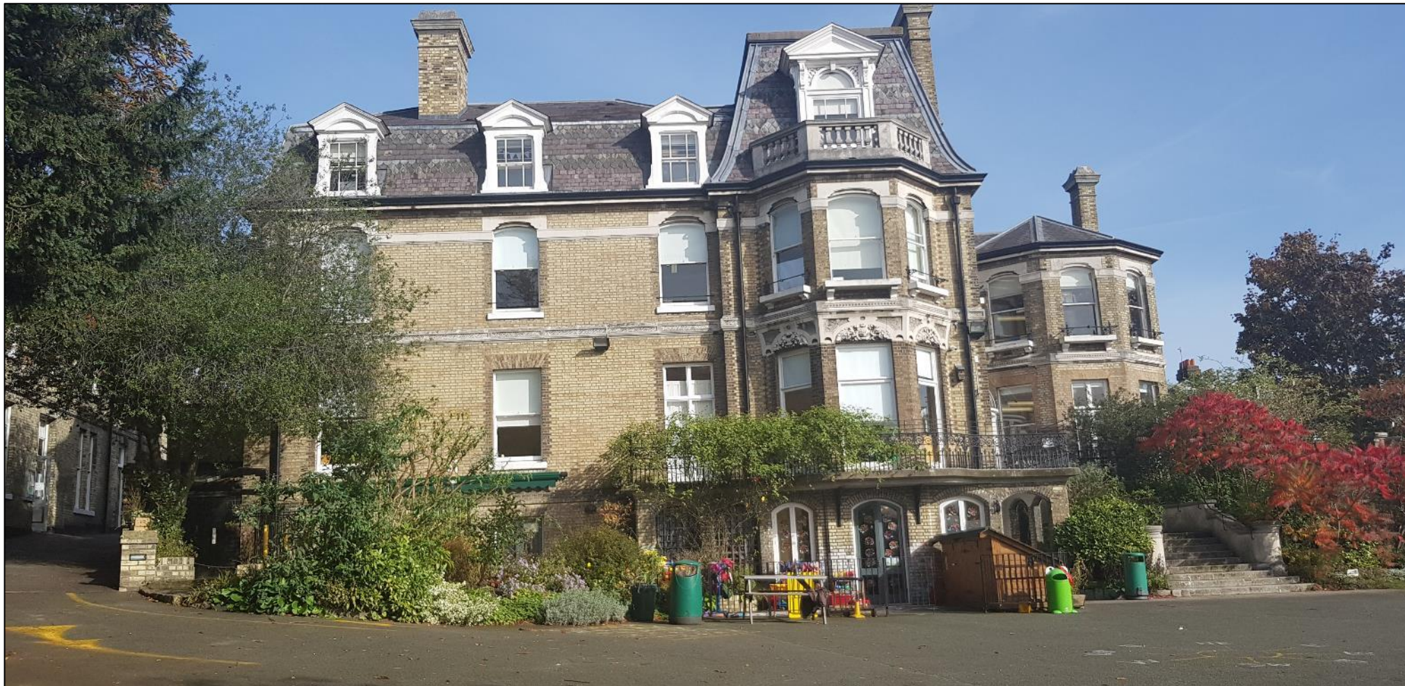
Photo 2: Looking north at the rear B1.
