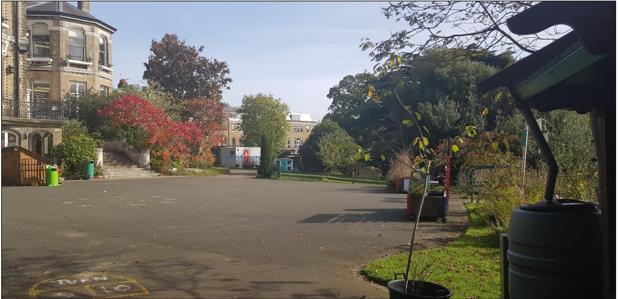
Photo 5: Looking east across the rear playground. This is the main area of the proposed works.
