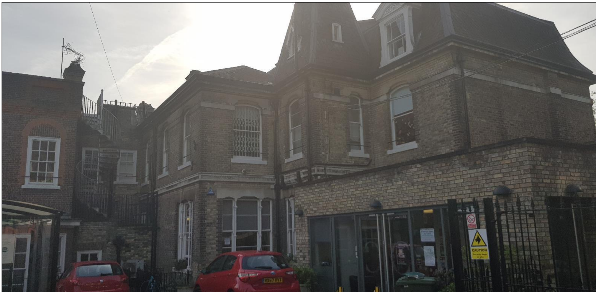
Photo 1: Looking south-west at the front of the main school building, B1.
