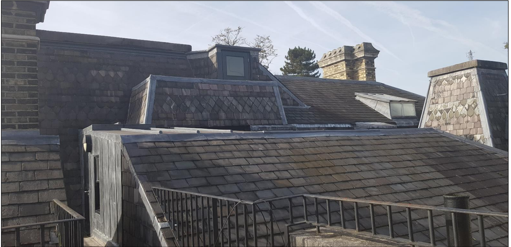
Photo 4: The roof of B1.
