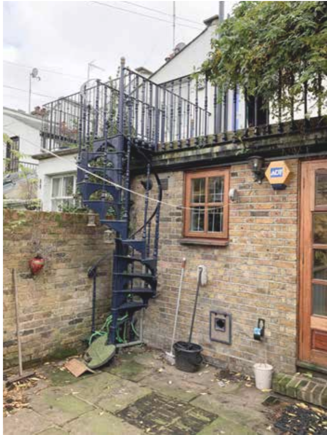
View of the existing extension wall and staircase
