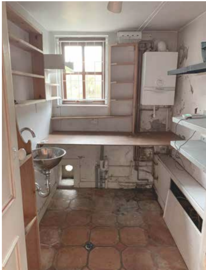
Ground Floor utility room
