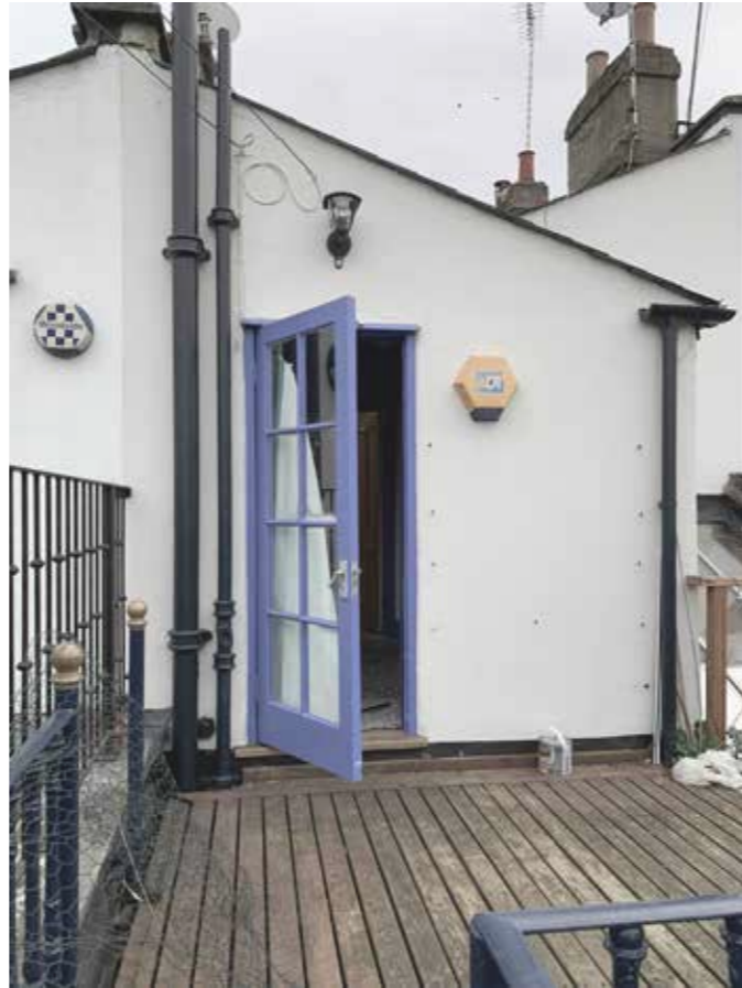
1st Floor Exterior Terrace
