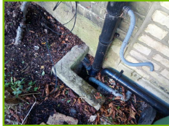
Fig 1.1: Combined waste gully 1
