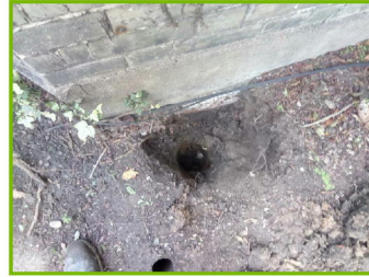
Fig 1.2: Internal view of trial hole
