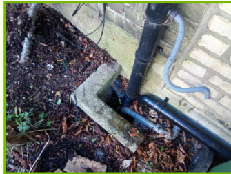
Fig 1.1: Combined waste gully 1
