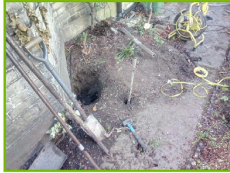
Fig 1.1: Carrying out trial hole
