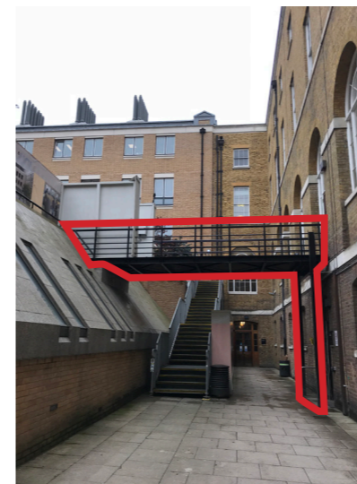
Bridge to be carefully removed.
