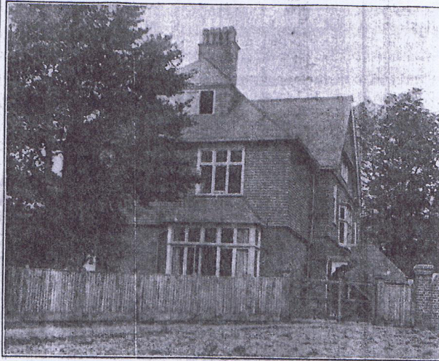
This house, built in 1892, is the residence of Mr. Walter Besant, the celebrated novelist.
