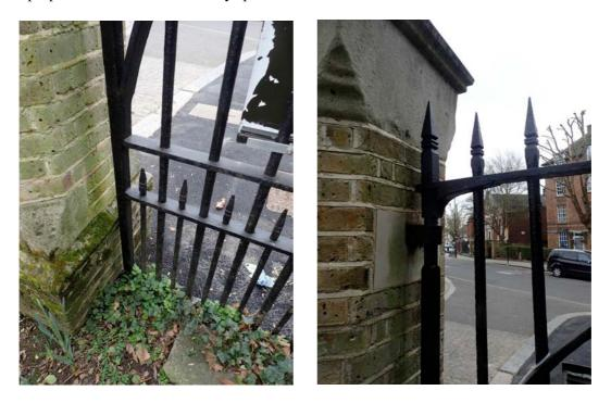
All of the proposed works will be carried out using traditional materials and building methods appropriate to an historic structure, including forged iron and steel work, reclaimed and matching bricks and new stonework laid and pointed in lime mortar and traditional natural materials for paving.
