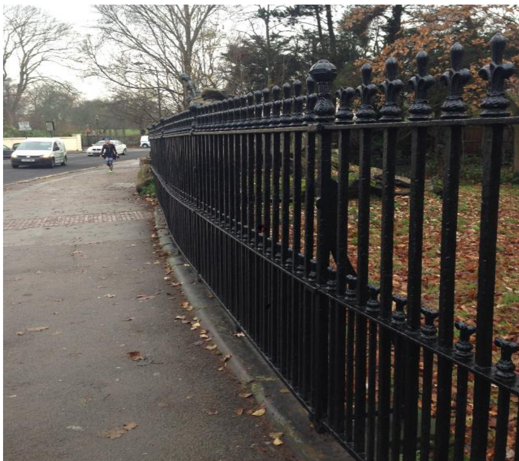
Photo 1: Garden Railings to Gloucester Gate Lodge.
