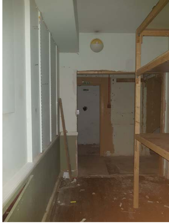
Photograph of existing Basement
