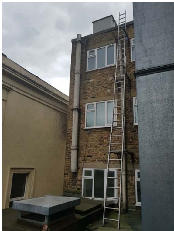
Photograph of rear Section of the Building
