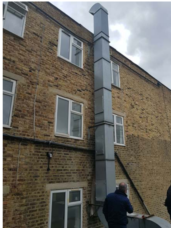
Photograph of rear Section of the Building
