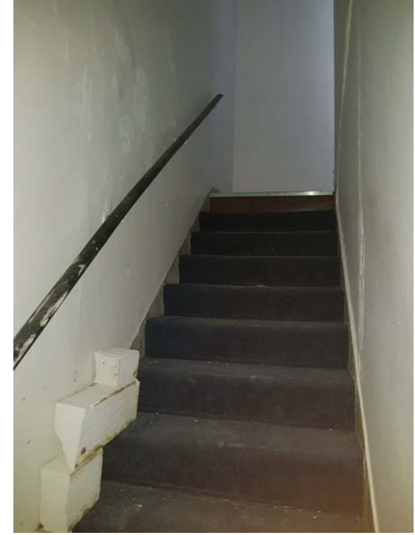
Photograph of Stairs to Ground Floor
