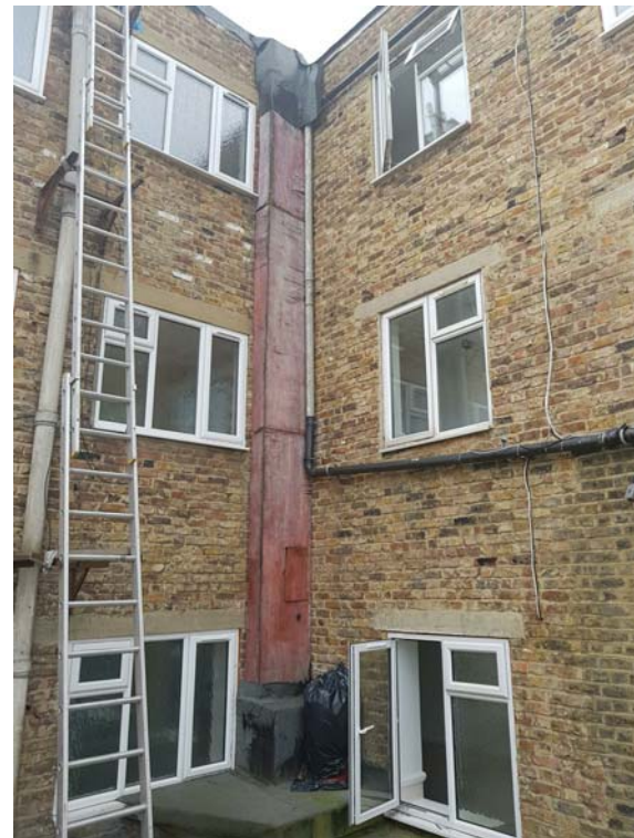
Photograph of rear Section of the Building
