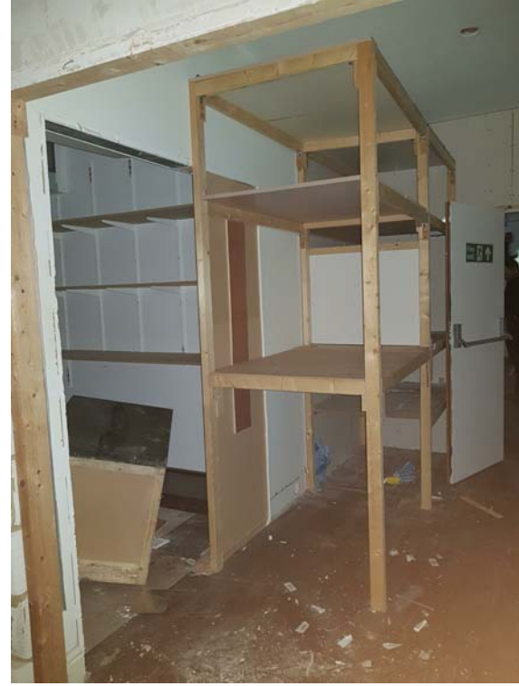
Photograph of existing Basement
