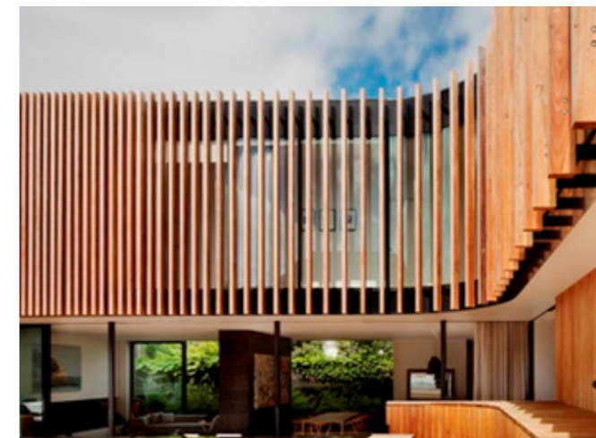
Vertical Timber Cladding With Glazing
