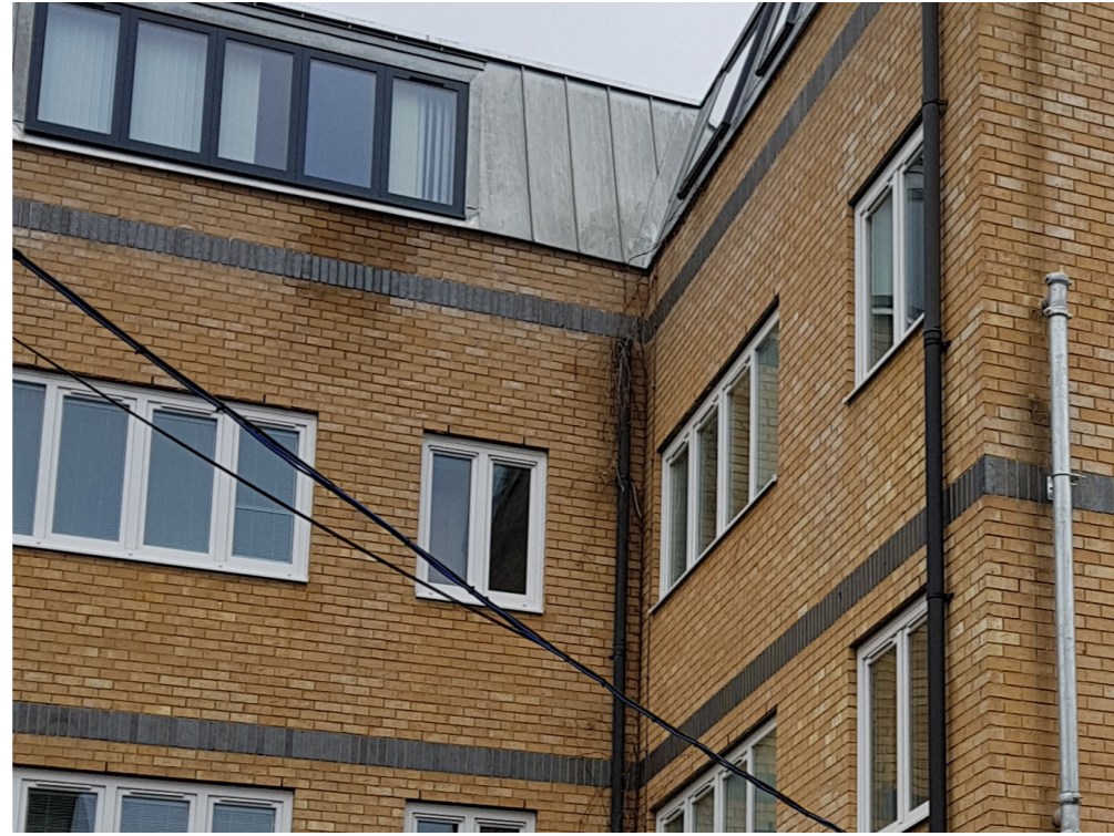
Existing Building: 73A Maygrove Road
