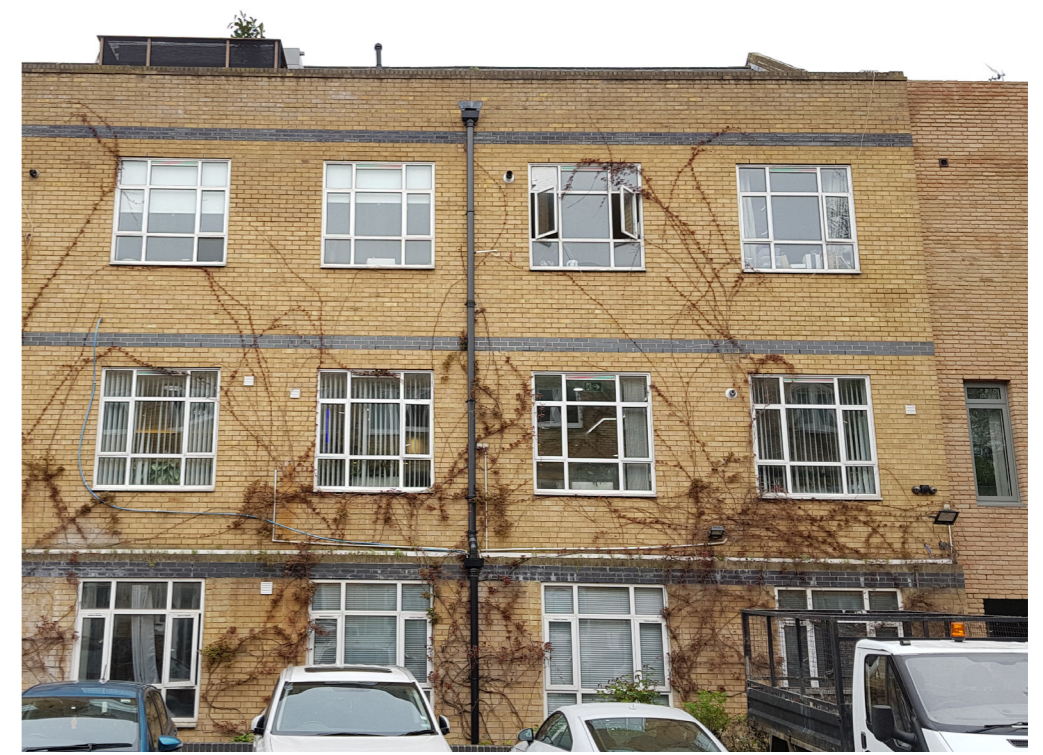
Existing Building: 73A Maygrove Road
