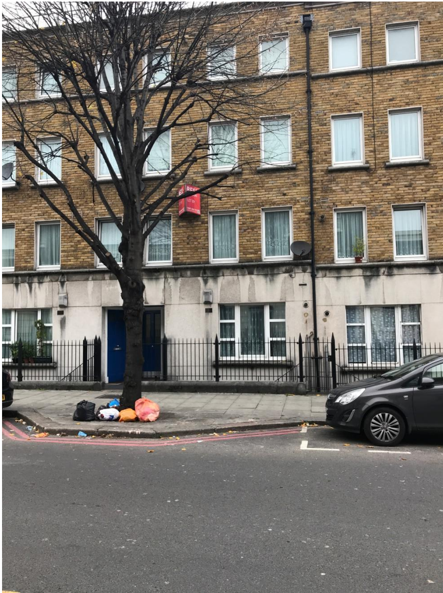
General View of front elevation
