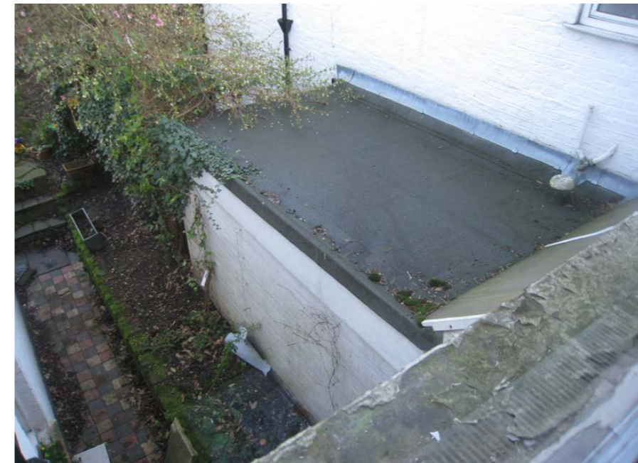
Side passage with No. 13 - View of neighbours side extension
