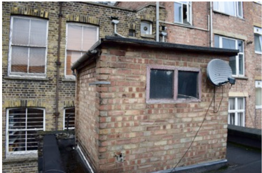
Drawing of c1950 showing proposed lavatory accommodation to be added to the flat roof at the rear of the building designs by Harold Quick, A.I.N.A.; (probably), the completed building. (Note asbestos construction)
