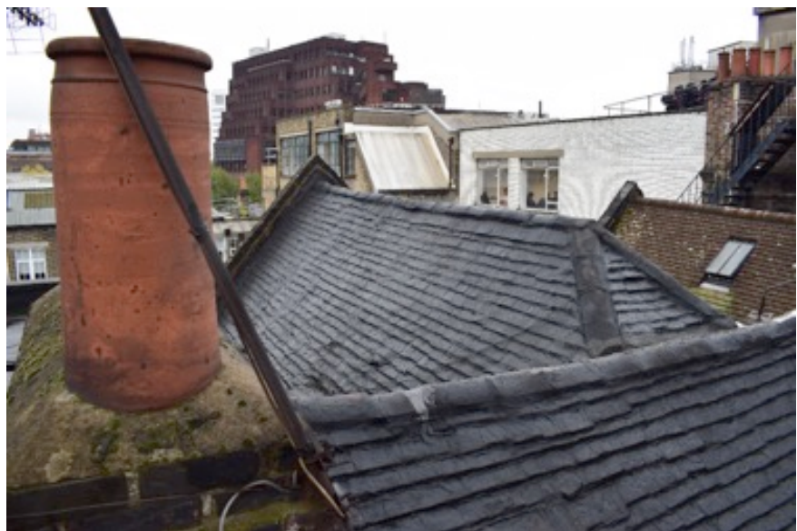
View of the neighbouring, hipped roofs of No.6 Denmark Street- still preserving the original (late 17thC) roof forms
