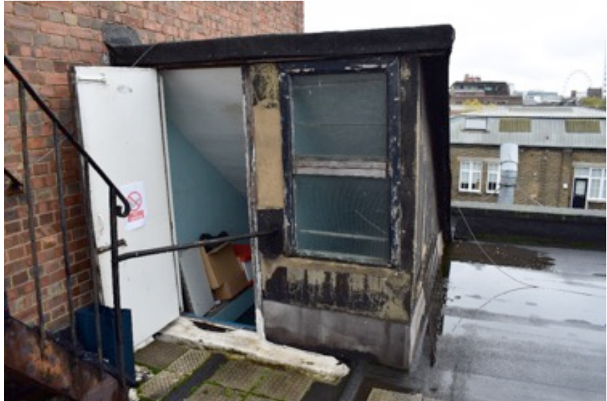
Enclosing structure around upper level of stairs; probably of early-mid-C20 date
