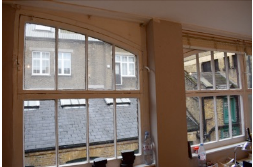
Views inside the three-storey late-Victorian workshop extension at the rear
