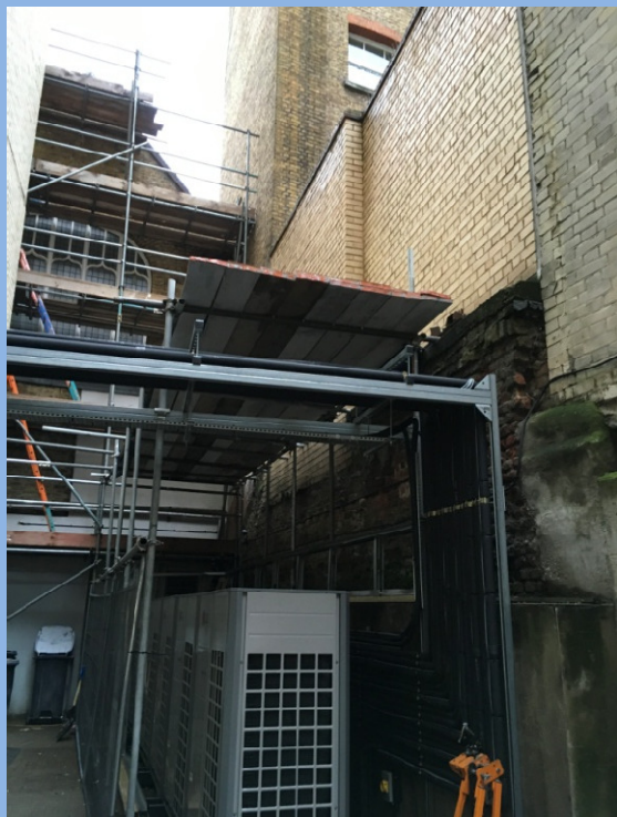
3 – units to rear access way. Units are obscured from view with high blank walls. These units are proposed to have acoustic enclosure built around them to provide noise attenuation.
