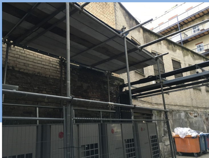
3 – units to rear access way. Units are obscured from view with high blank walls. These units are proposed to have acoustic enclosure built around them to provide noise attenuation.
