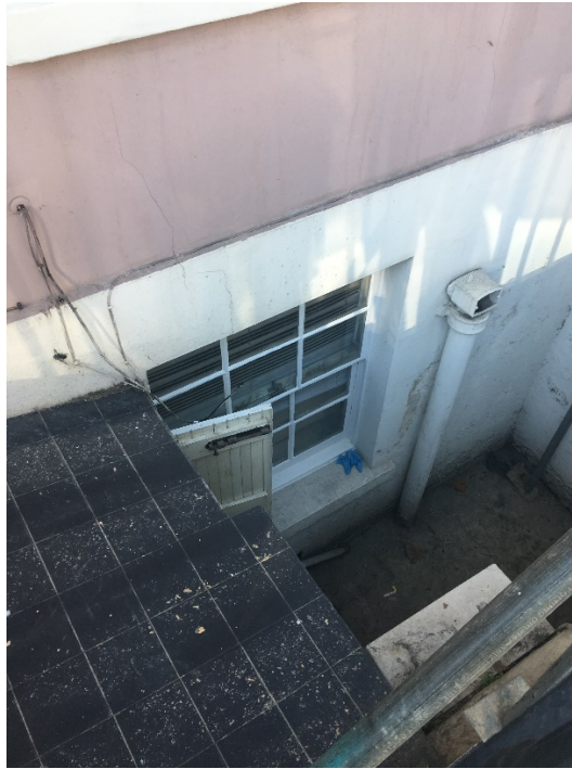
Photograph 15.1 – Damaged render on front elevation
