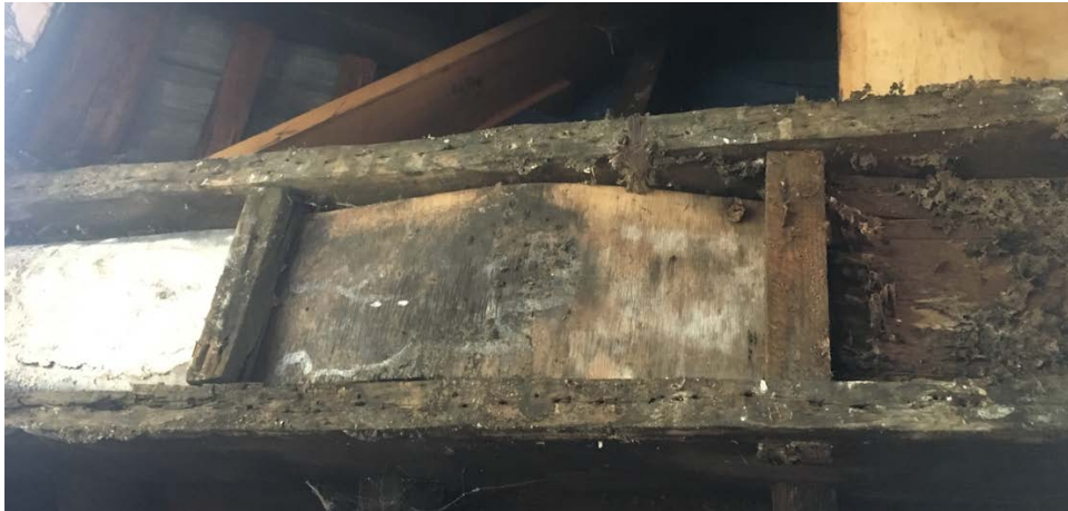
Photograph 12.1 – Rotten timbers and leaking leadwork
