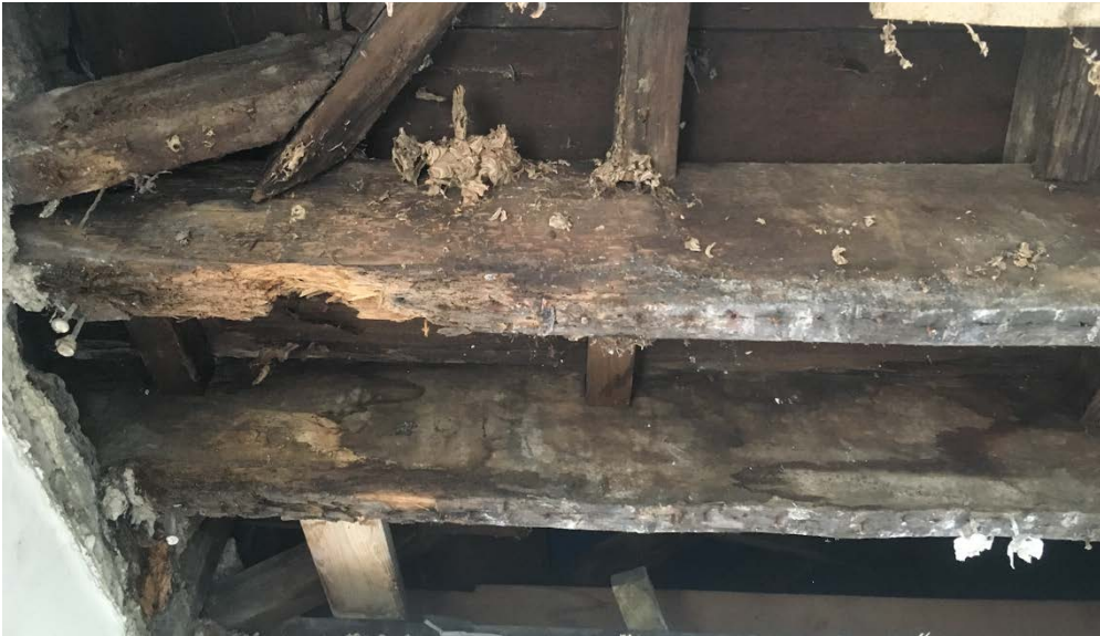
Photograph 12.2 – Rotten timbers where new supports were attached either side
