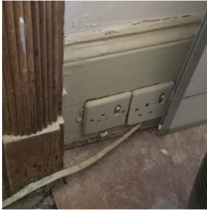
Photograph 20.1 – sockets which has been removed and have left holes within the skirting board.
