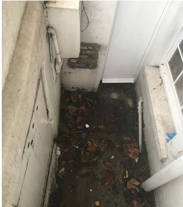
Photograph 17.1 – Hole from previous extractor which has been repaired.
