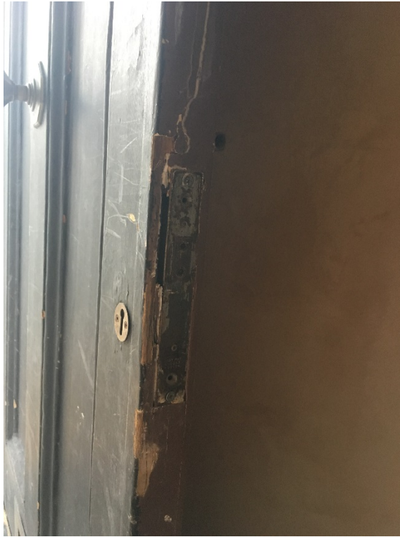
Photograph 9.3 - Existing door showing damage and poor repairs
