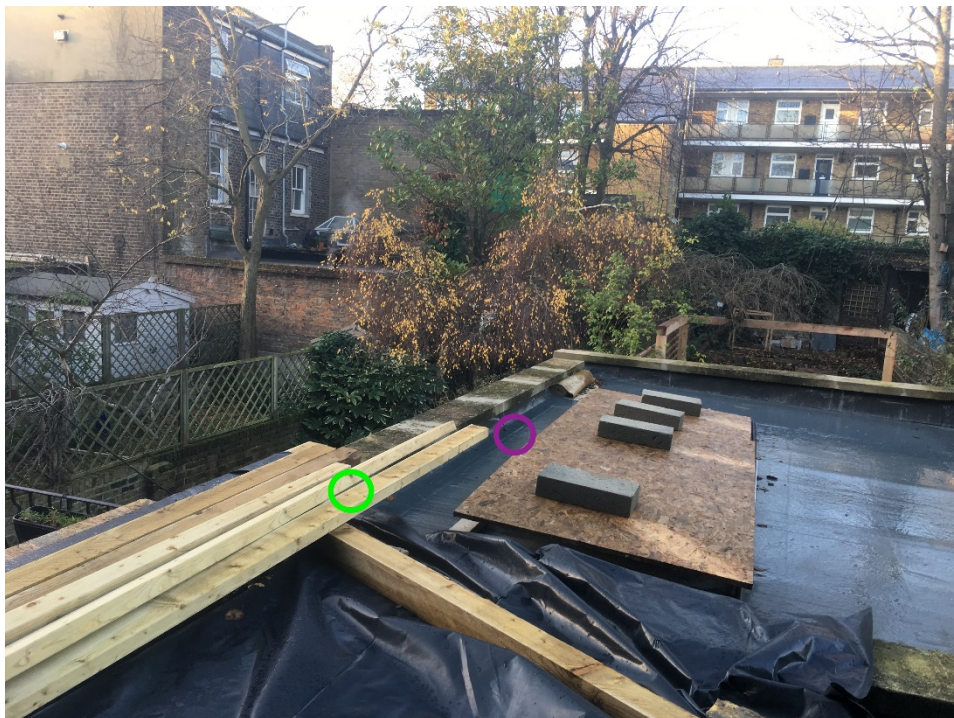
Photograph 7.1 – preferred location of extractor (purple) compared to alternative (green)
