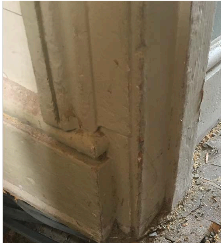
Photograph 5.4 - Showing hallway door mitred over original skirting which was corrected by removing the door
