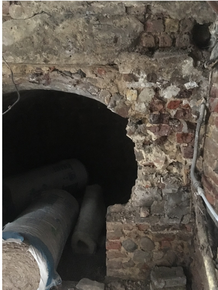
Photograph 2.2 – Damaged entrance to newly discovered internal vault
