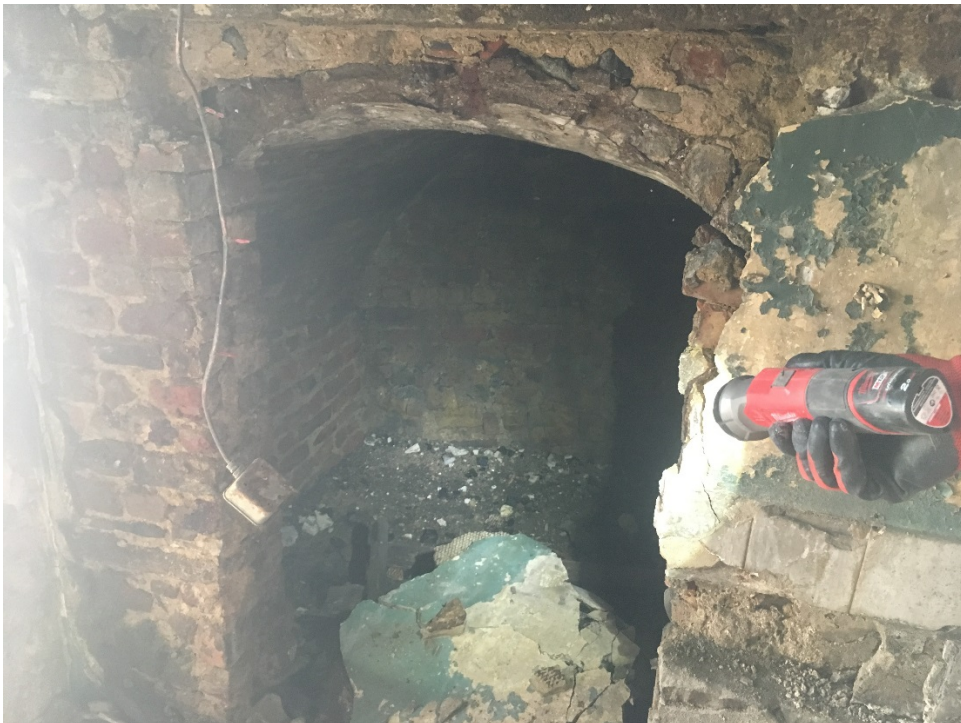
Photograph 1.2 – Newly discovered internal vault
