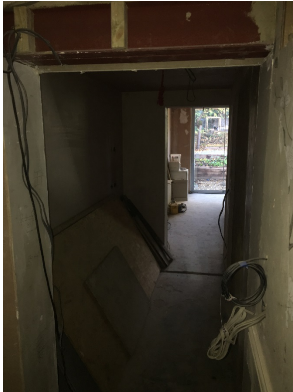
Photograph 3.2 – Relocated hallway doorway
