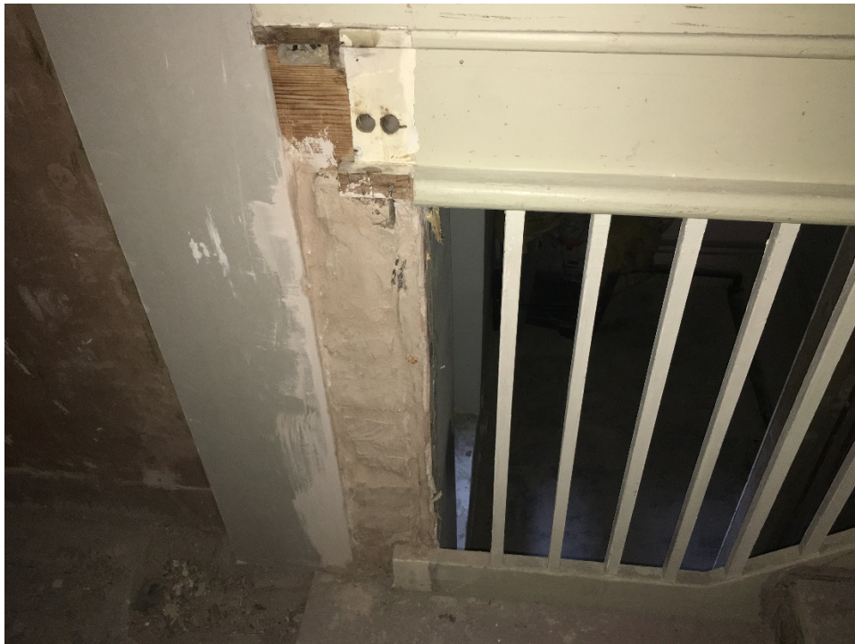
Photograph 3.1 – Relocated hallway doorway
