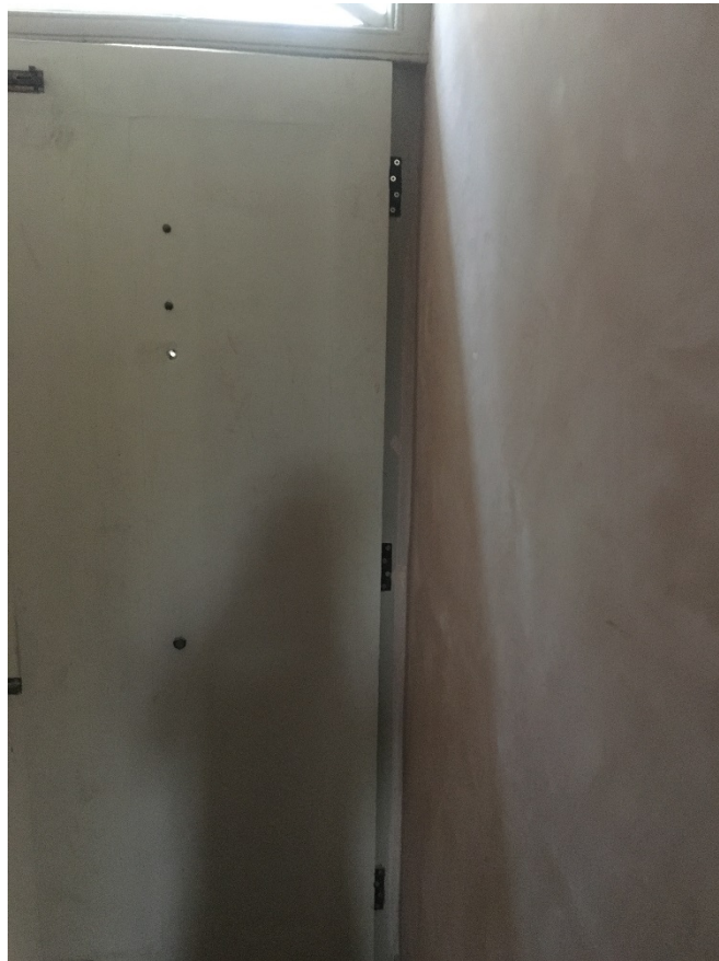
Photograph 9.4 – Existing door showing insecure hinges
