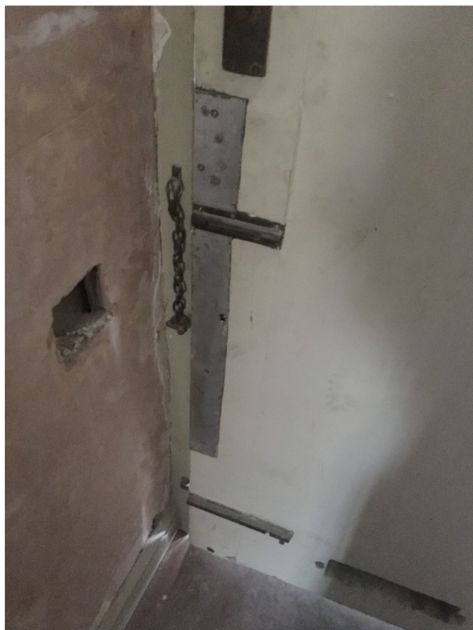
Photograph 9.2 – Existing door showing damage and poor repairs
