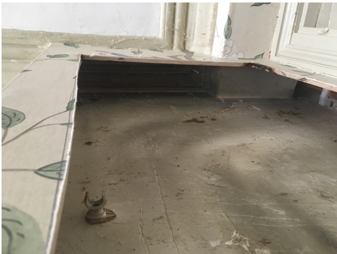
Photograph 5.3 – Hallway door prior to removal showing original cornice being uncovered
