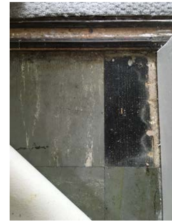
Existing photos showing broken, missing and uneven vinyl tiles
