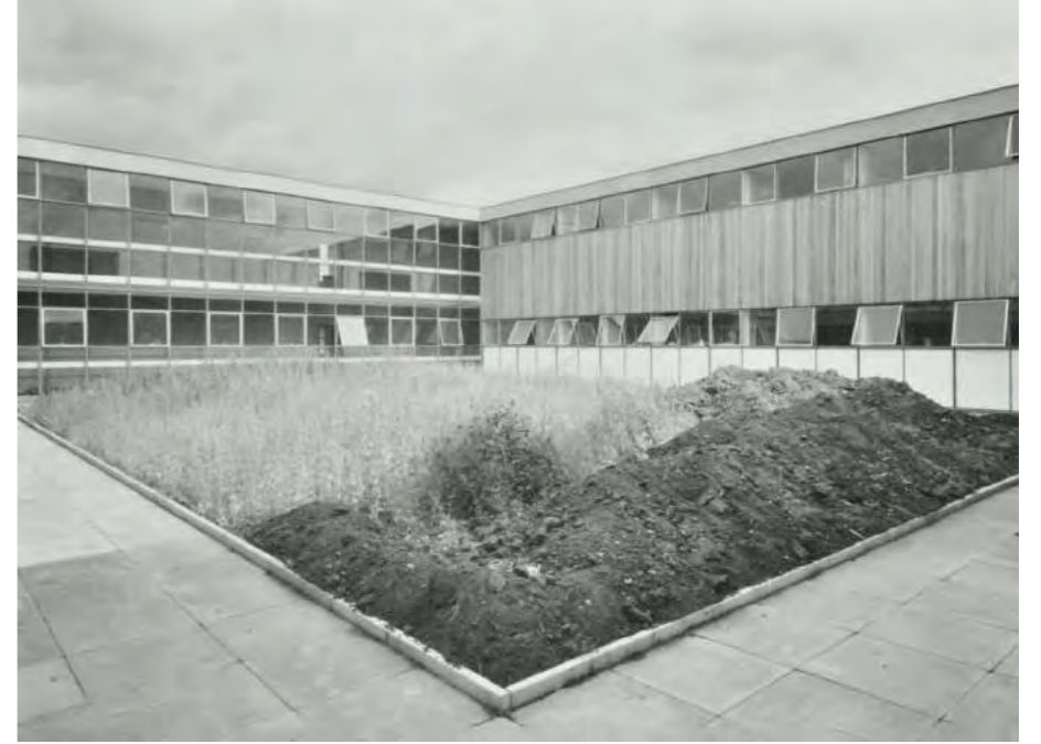
1988: Photograph of school building, view of East internal courtyard
