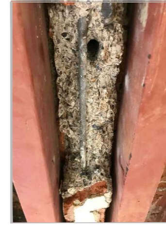
Pl2: STEEL SAMPLE LOCATION TO SOFFIT OF RIBS AFTER EXTRACTION
