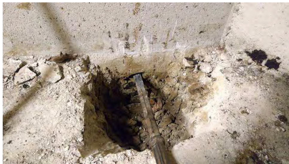
TP04 (foundation inspection pit).
