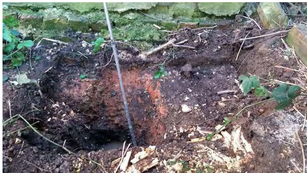
TP01 (foundation inspection pit).
