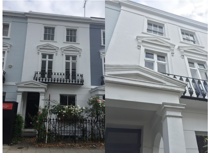
The highlight of 4 Chalcot Crescent's historical merit is found in its front elevation & unusual portico structure.
