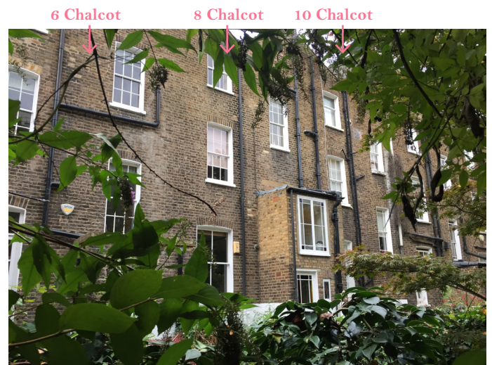
The view over the garden wall of 4 Chalcot Crescent.
