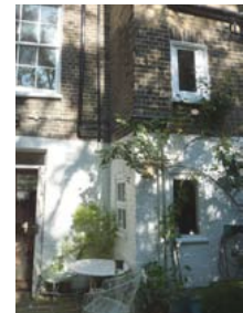
18 Chalcot Crescent closet wing windows
