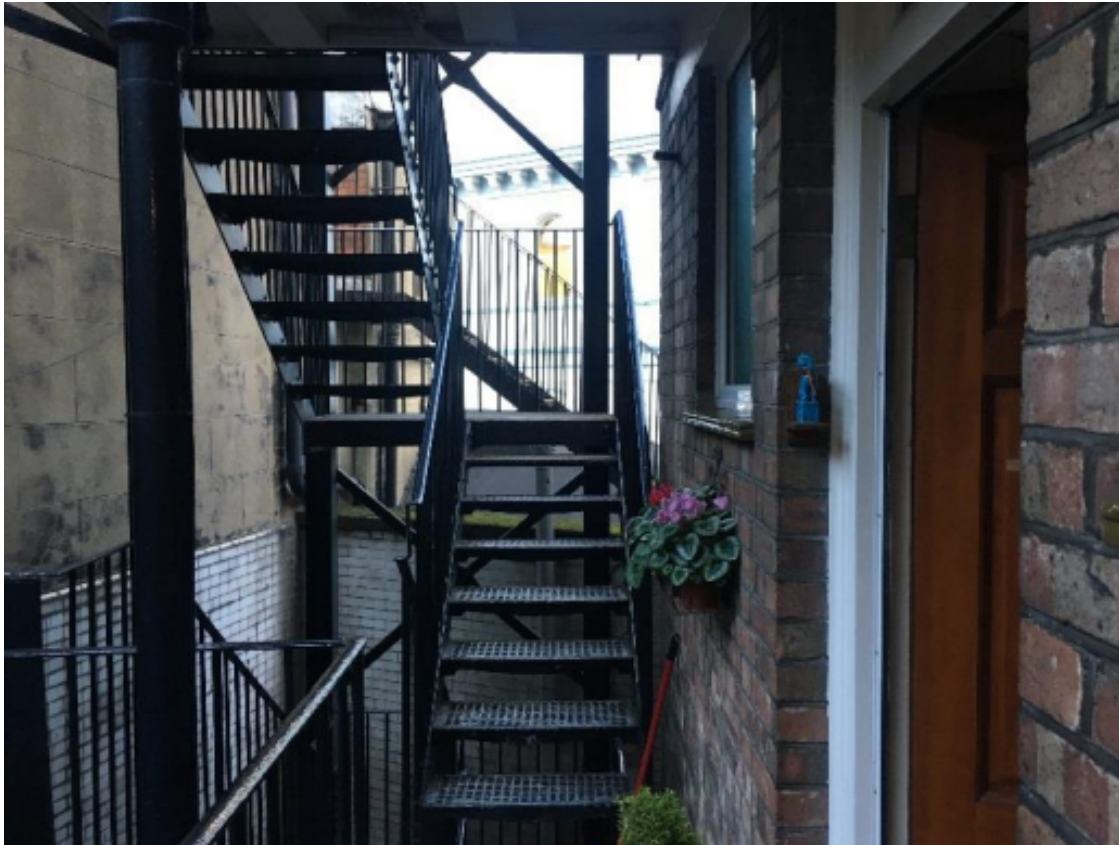
Photo 3: rear lightwell staircase showing location of proposed ducting (to the left hand side of the stairwell). Photograph provided by objector.
