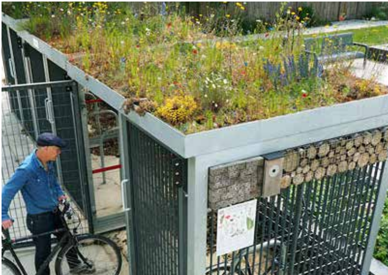
Bin Shelter roof to accommodate 150mm of topsoil to receive meadow seed planting
