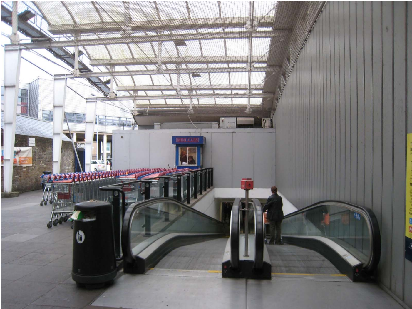
View 20. The travelator that links the store to the underground car park is an important feature. The slight adoption of the wheels of the shopping trolley made it possible to anchor them to the moving traveller so that it is easy to move large loads from one level to another. This device revolutionised the design of supermarkets by advancing the notion of the supermarket as a multi-use building.
