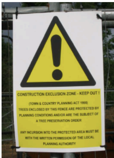
Figure 3 – Example of suitable warning sign affixed to protective barrier
