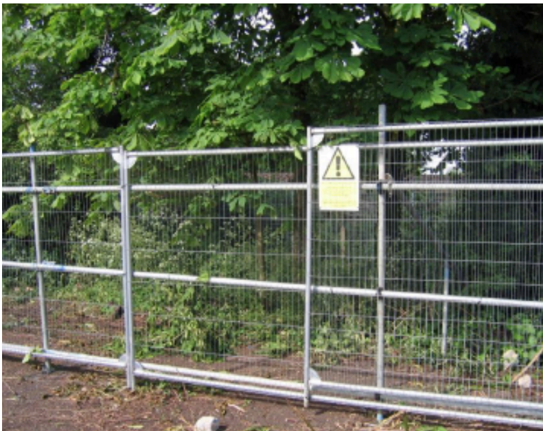
Figure 3 – Example of suitable warning sign affixed to protective barrier
