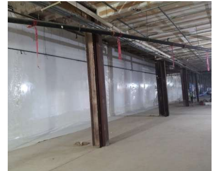
Figure 13 - Temporary Dust Partition on site
