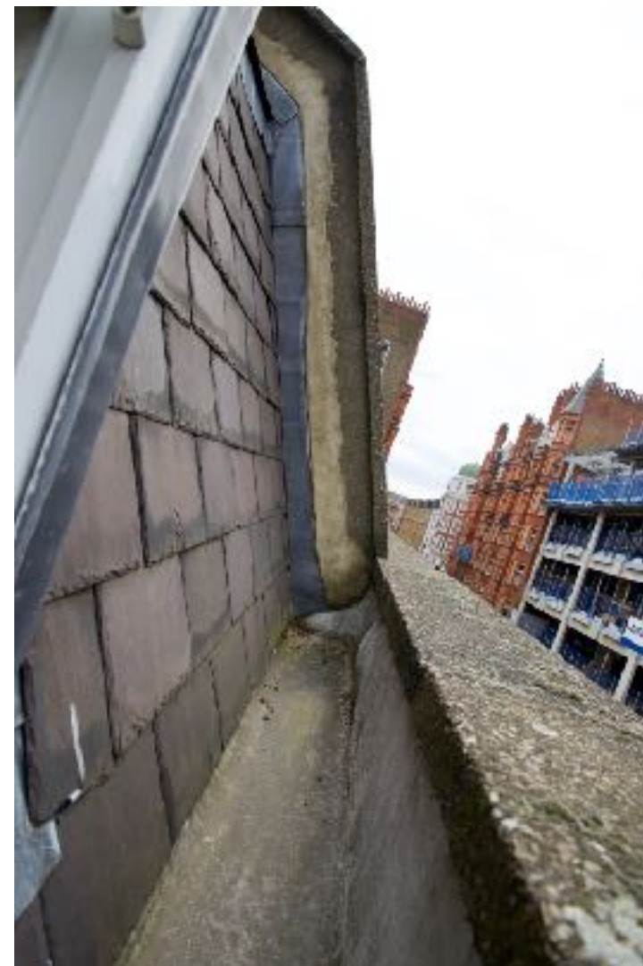
Pic 11 Parapet gutter and upsand wall with patchy render
