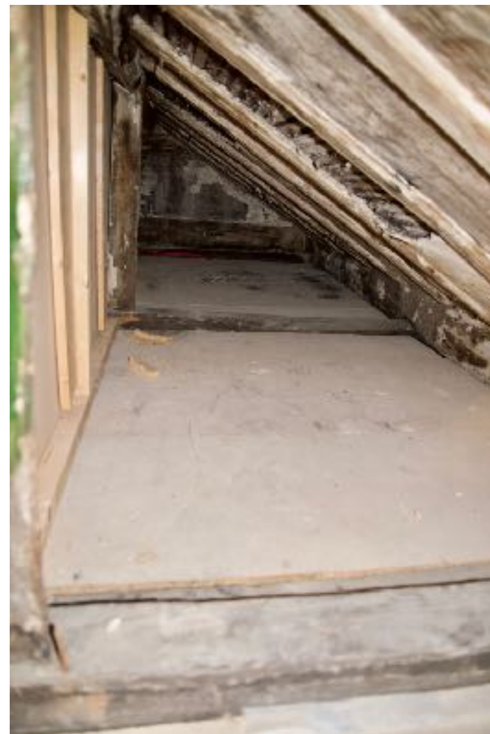
Pic 13 View of loft space over 62 Huntley Street indicating stained roof timbers
