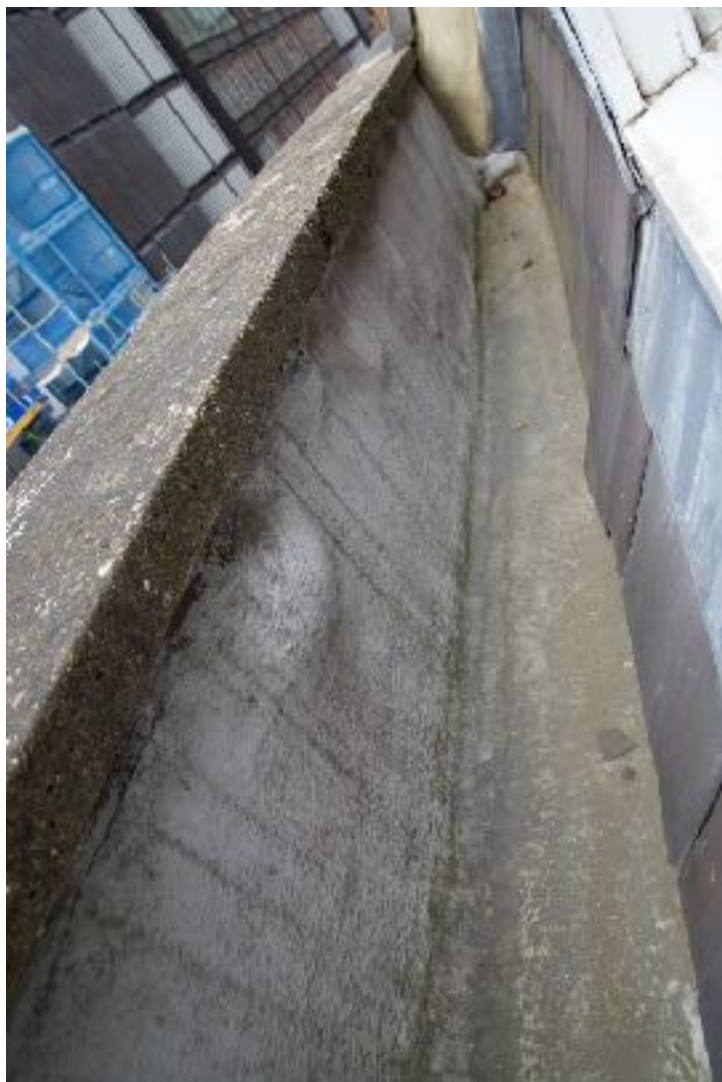
Pic 10 View of parapet gutter indicating slumping asphalt
