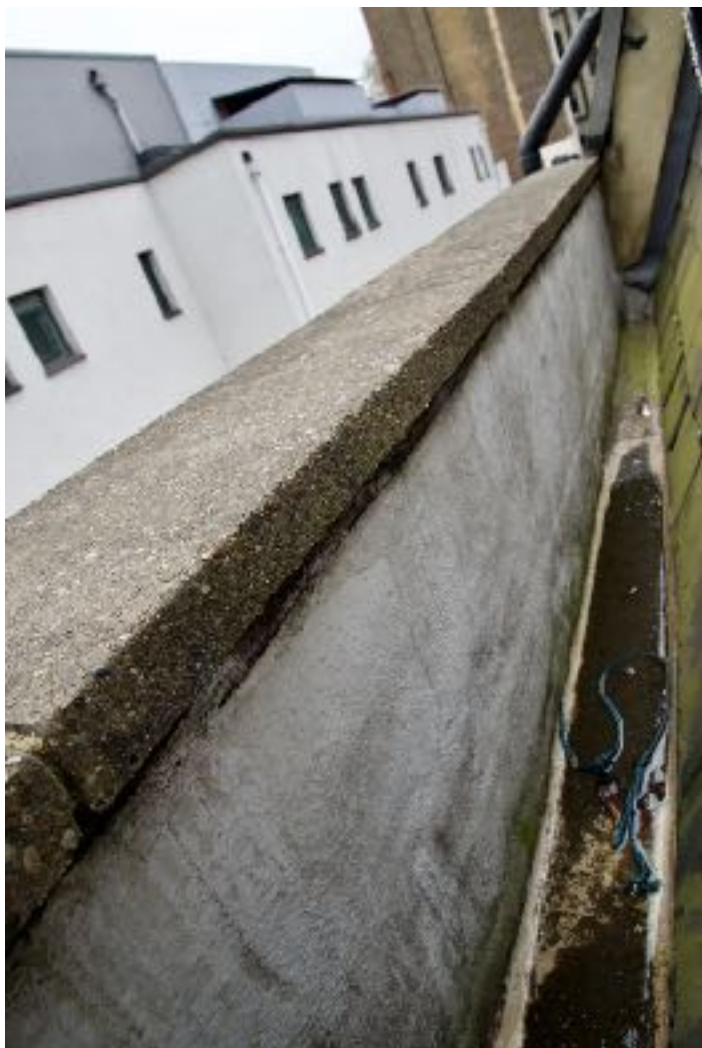
Pic 12 Standing water noted on one parapet gutter
