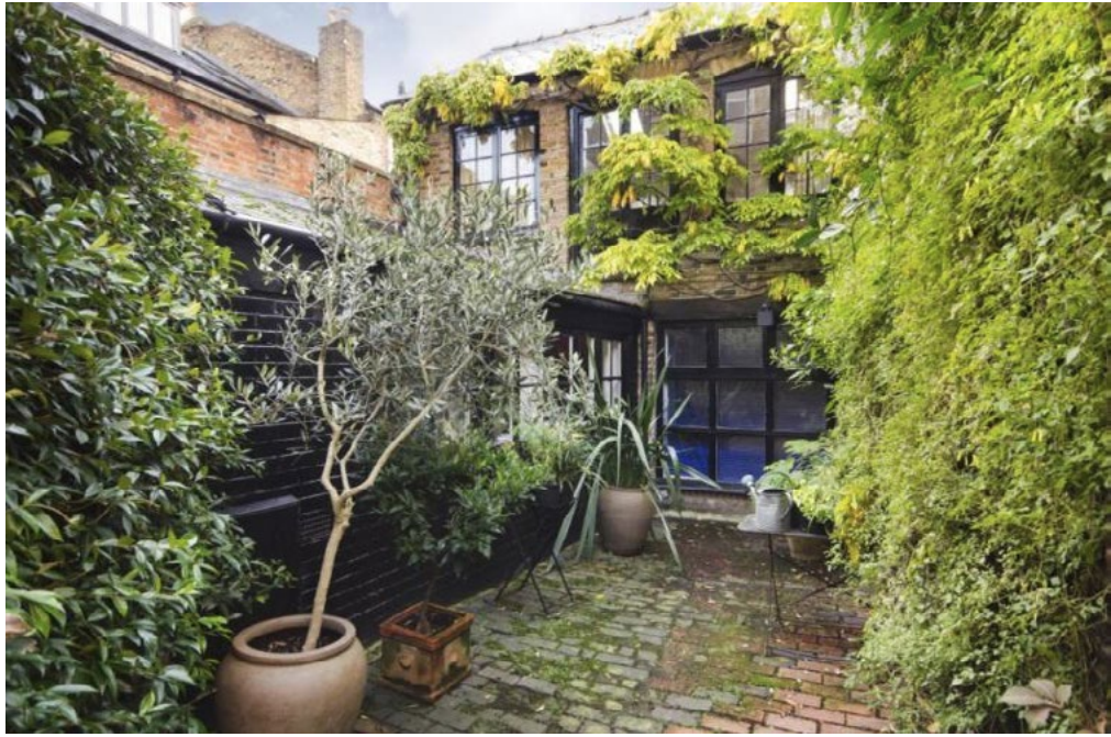
The existing yard with the main studio building and lean-to (on the left)
